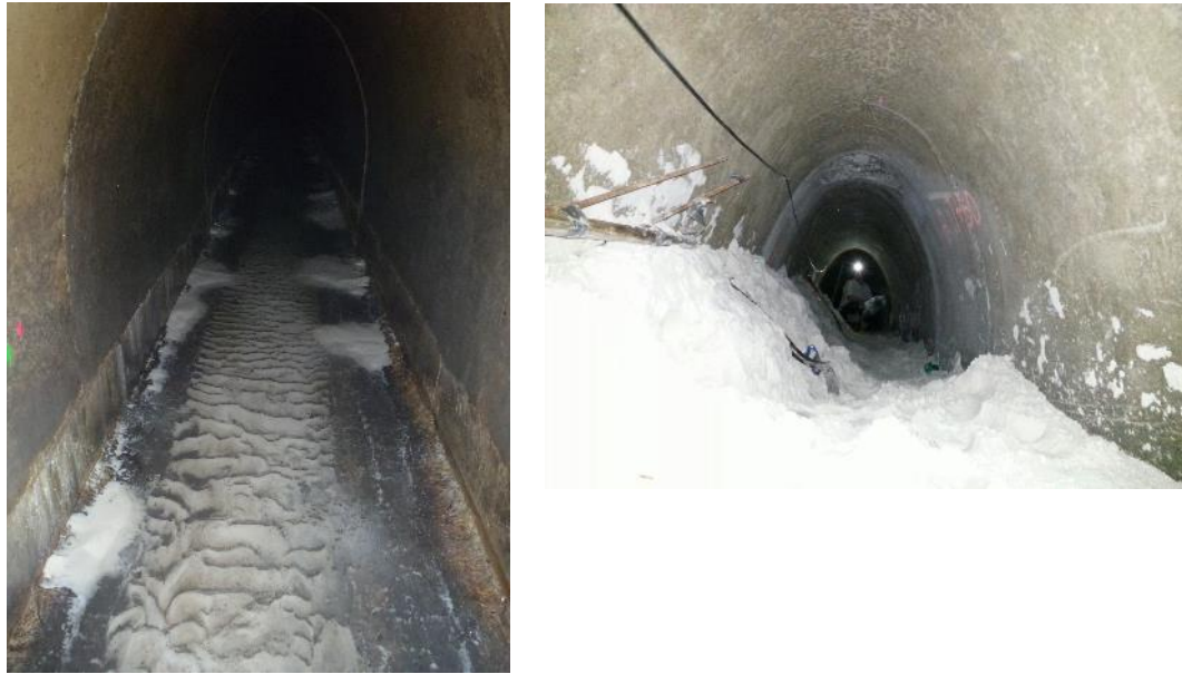
Figure 5.16 – Photographs of Sand in Tunnel
