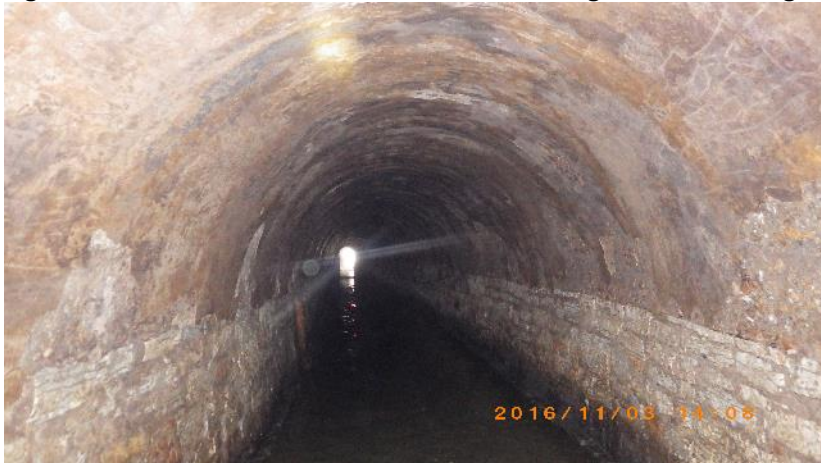
Figure 3.1 – 2 nd Street South Tunnel Above Convergence with Chicago Avenue Tunnel
