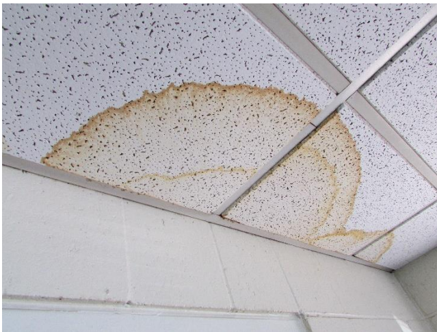
Rm 116 – Office – Water-Stained Ceiling Tiles
