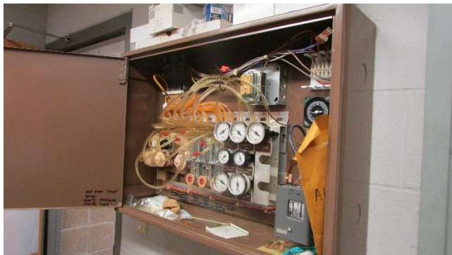
Rm 144 – Storage – Antiquated Pneumatic Controls
