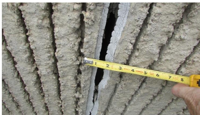
Example Of Recaulking Needed in East Side Exterior
