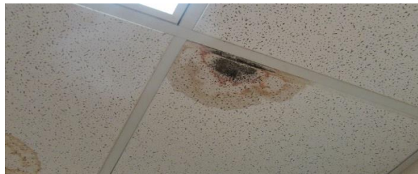
Rm 120 – Roll Call – Water-Stained Ceiling Tile
