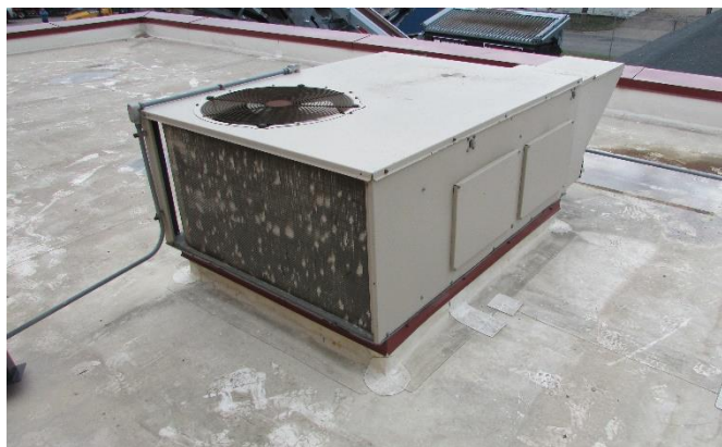
Hail Damage Visible on RTU's
