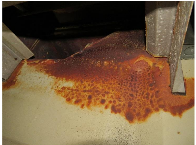
Rm 119 – Work Room – Furnace Corrosion
