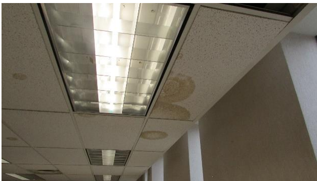
3 rd Floor Open Office – Water-Stained Tiles
