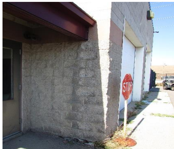
Split Face Block Erosion from Roof Water
