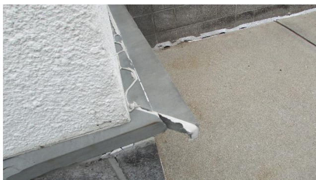
Southside - Exterior Stone Trim Piece Requires Repair
