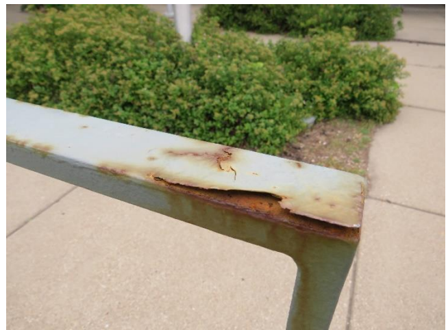
Northwest Entrance – Peeling Paint from Railing
