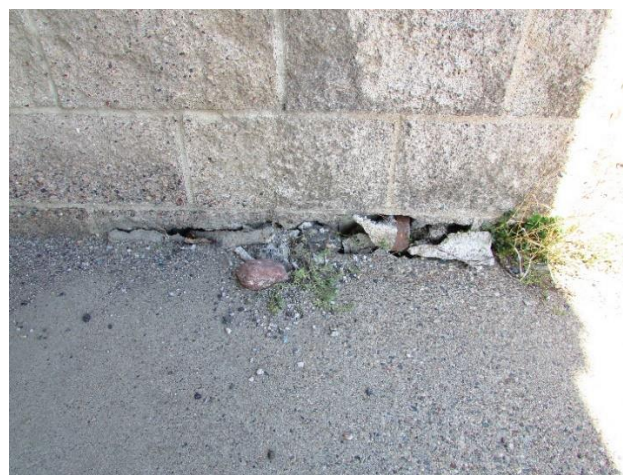
Block Deterioration at Base Near Main Entrance
