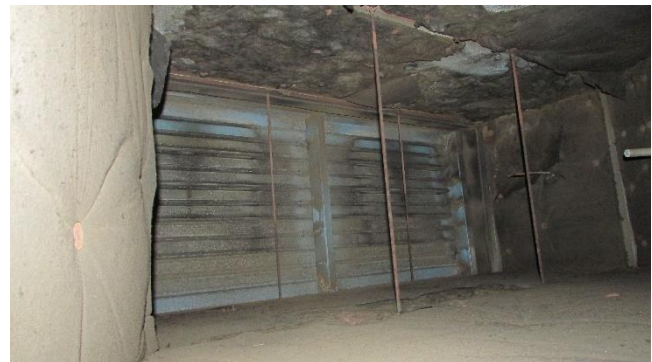
N Mech Penthse – Range MUA Unit – Dirty / Interior
