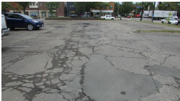
Cracks/Deterioration/Ponding in Asphalt Parking Lot
