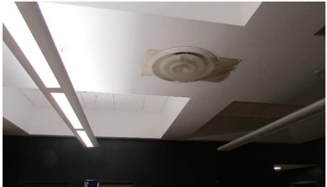
Plastic Covering Supply Diffuser On 2 nd Floor Open Office
