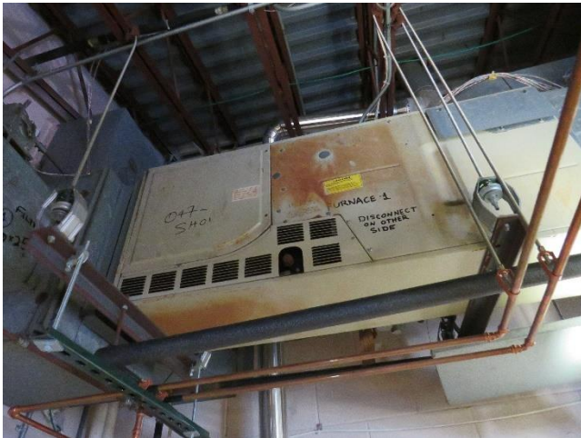
Rm 119 – Work Room – Furnace Deterioration/Corrosion
