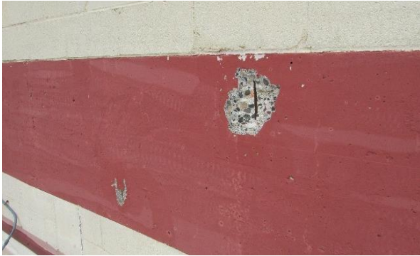
Damage On Exterior of Building
