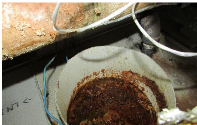
POR: Bucket Used for Hot Water Leak Collection
