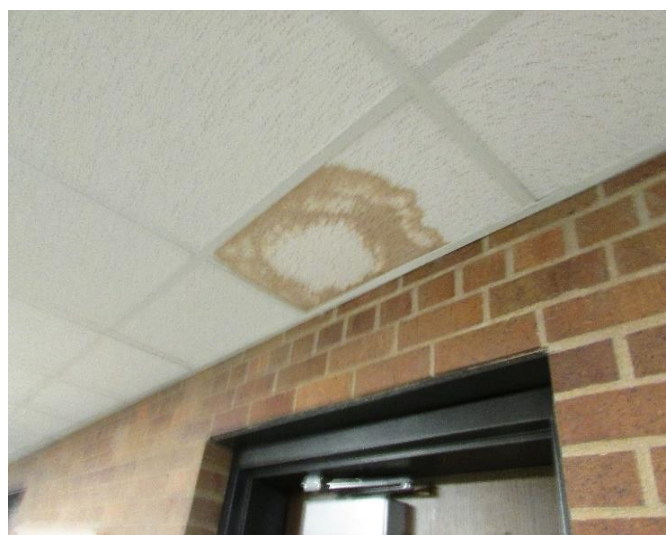
Rm 134 – N Hallway – Water Stained Ceiling Tiles
