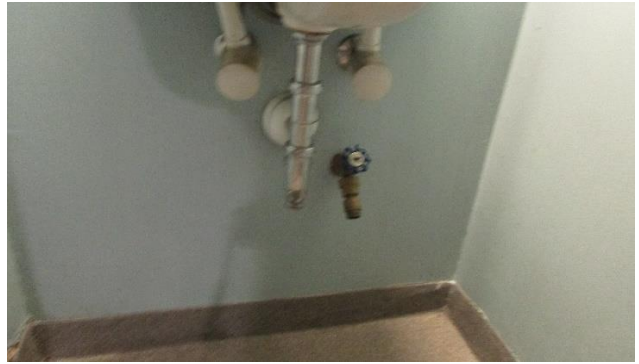
Lack of Pipe Wrap in Accessible Labeled Restroom
