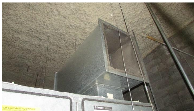
Traffic: Return Air Duct – Drawing Air from Above Ceiling
