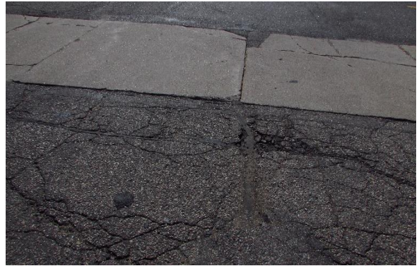
Cracks/Deterioration in Asphalt Parking Lot
