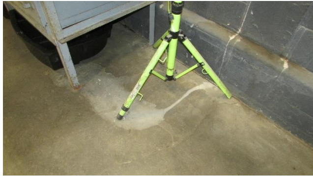
Evidence of Roof Leak Located on East Side
