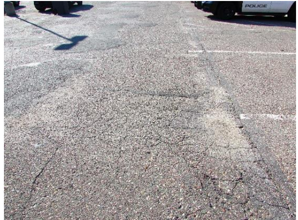
Cracks/Deterioration in Asphalt Parking Lot
