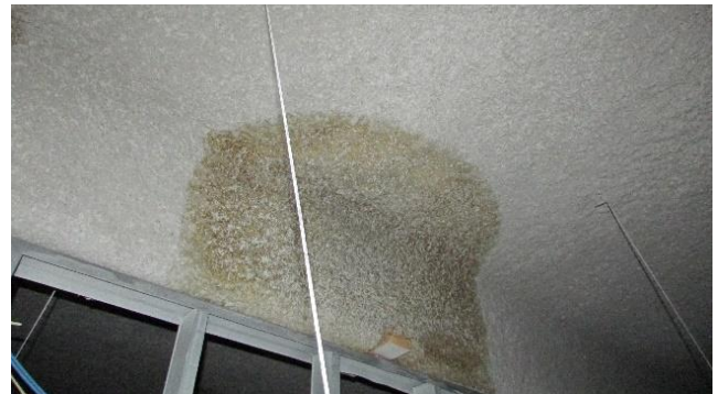
Rm 308 – Water Damage Above Ceiling Tiles
