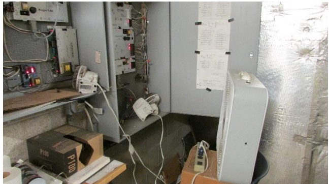
Rm B11A – Multiple Fans Cooling to Control System
