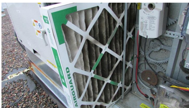
5 Ton Aeon Rooftop Unit (Pre-Filter) Needs Changing
