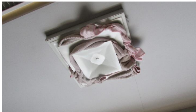
Rags Have Been Stuffed into Supply Air Diff on 2 nd Flr
