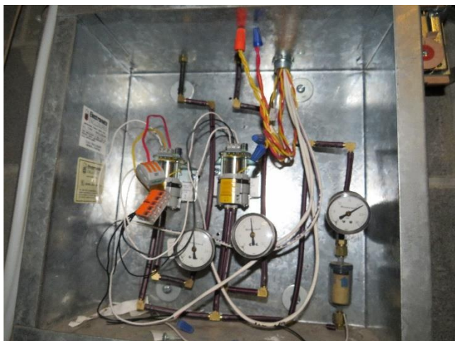
Rm 138 – Utility - Archaic Pneumatic Temp Controls
