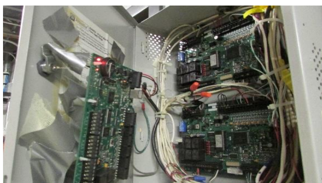
Rm 110—Telecom – Duct Tape Used in Panel
