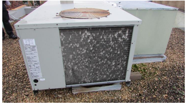
RTU-3 Condensing Coil Hail Damage
