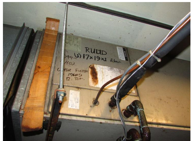
Rm 109 – Mechanical – Cardboard Used on Filter Bank
