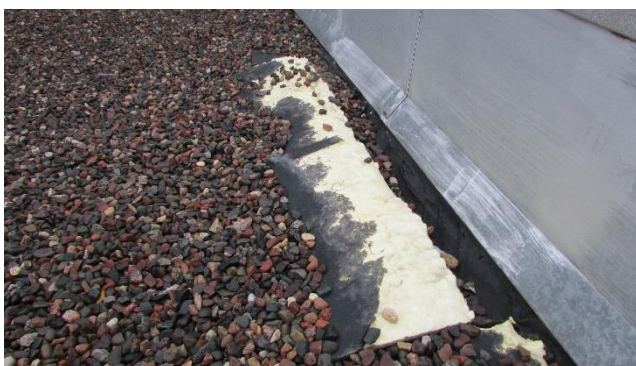
Exposed Insulation on the Roof
