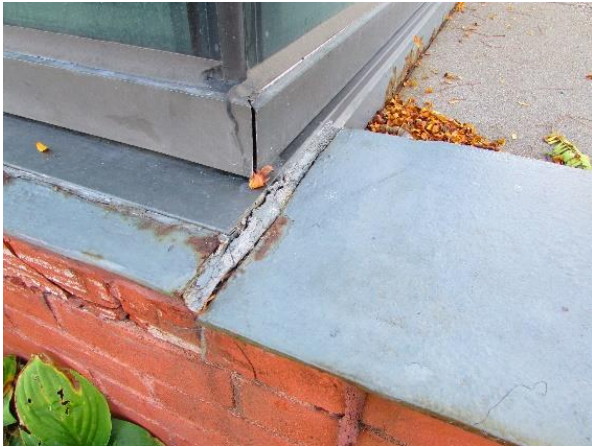
NW Failing Caulk Joint, Deteriorated Brick & Window Jt
