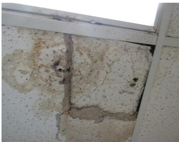
Rm 17 - Comm. Rm – Signif. Water Damaged Ceiling Tile
