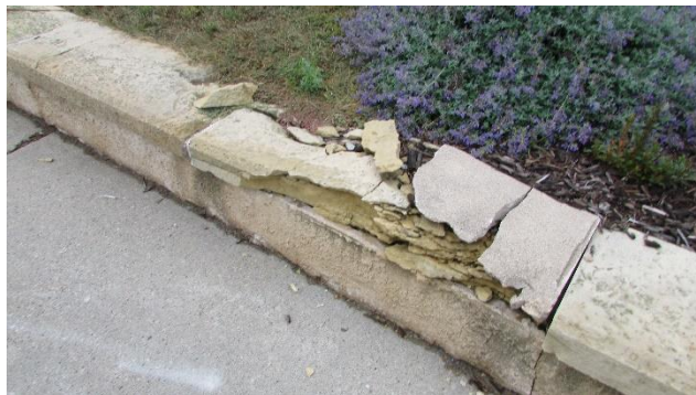
Retaining Wall on Eastside is Crumbling
