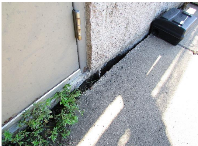
SW Corner, Drainage is Towards Building
