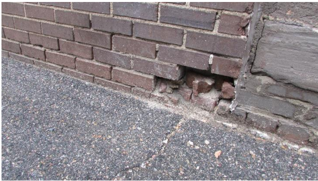
Exterior Brick (Eastside) Needs to Be Repaired
