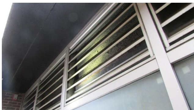
Plugged Outdoor Air Intake for Garage Make-Up Unit
