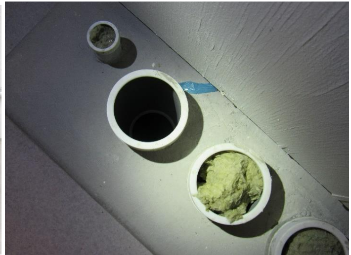
Lack Of Fire Stopping Around Elements in Elec/Telecom Rooms (Photos From 9 th Floor Elec/Telecom Rooms)
