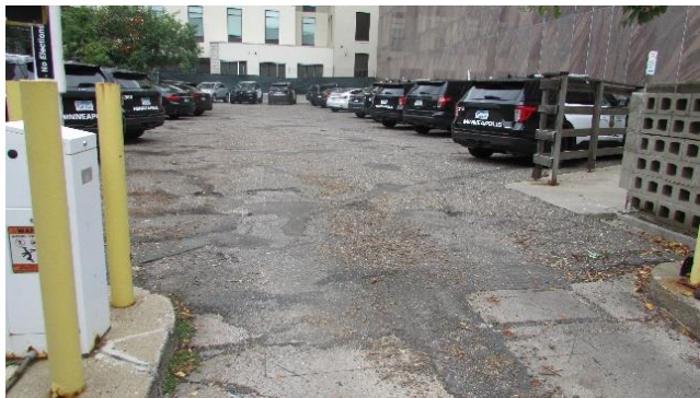
Parking Lot Cracking/Potholes/Deterioration
