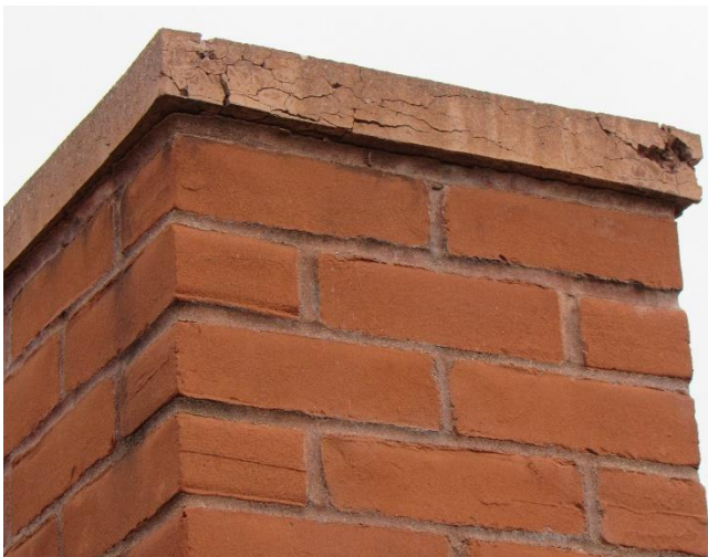
SW Brick Column (Vehicle Ent) – Crumbling Capstone
