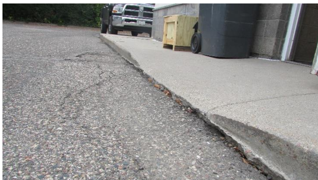
Approx. 1" Gap Between Asphalt & Sidewalk Ramp
