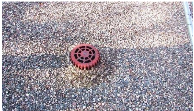
Roof Drains Need to have Debris Remove
