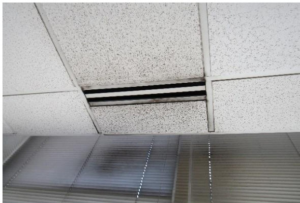
Traffic: Return Air Causing Dirt on Blinds
