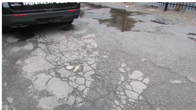
Cracks/Deterioration in Asphalt Parking Lot
