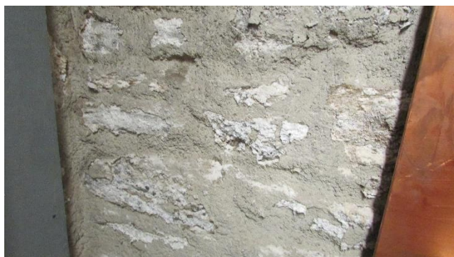
Rm 001 – Mech Rm – Foundation Surface Deterioration
