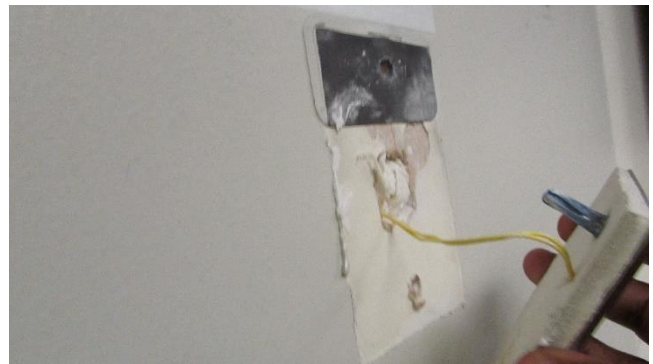
Rm 113 – Shift Office – Reattach Thermostat
