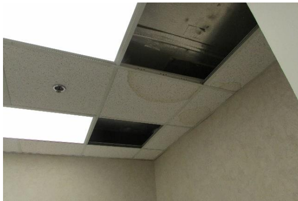
POR: Water-Stained Ceiling Tiles
