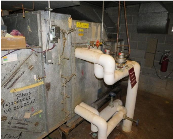
Multiple AHU's Are Past Expected Useful Life
