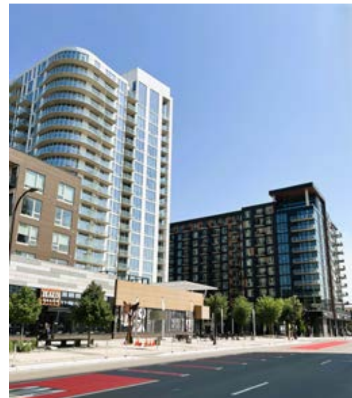
In this Transit 30 built form overlay district location, there are no individual building size limits for this PUD.
