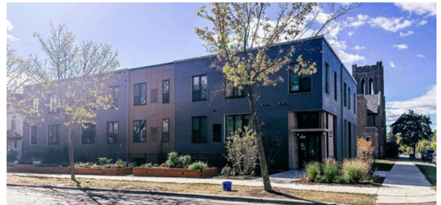
In this adaptive reuse and new construction project, part of a building that was first built as a church (in the background) was turned into apartments. The church still uses some of the space, but a new apartment building (in the front) was built where its big parking lot used to be.
