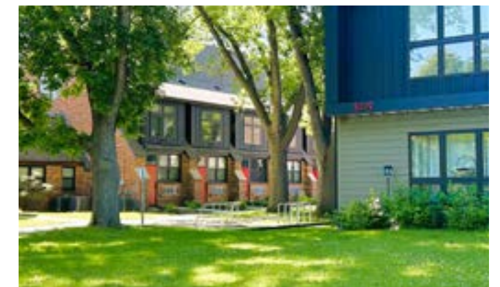
The original sanctuary (left) was converted into walk-up units with loft units above.
