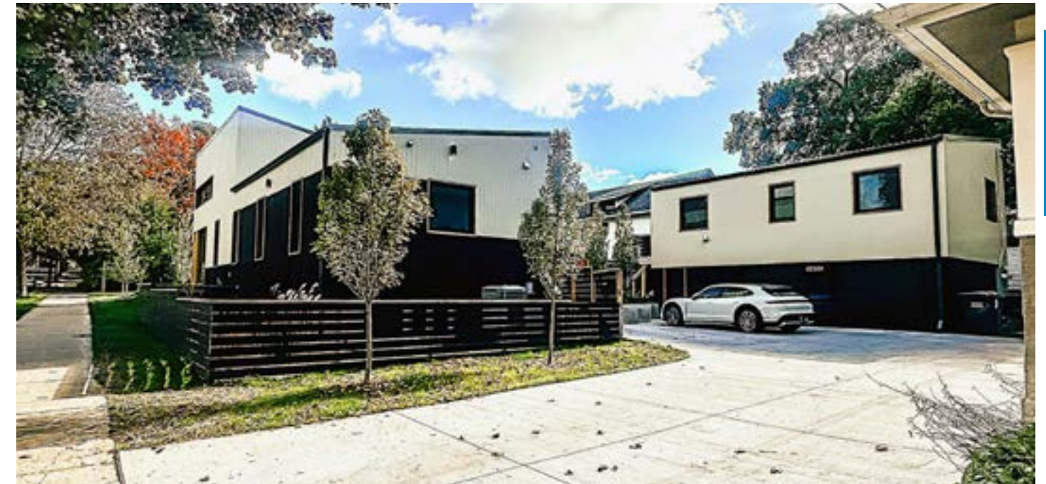
A detached accessory dwelling unit (right) contains living space above a garage for this new single-family dwelling (left).
