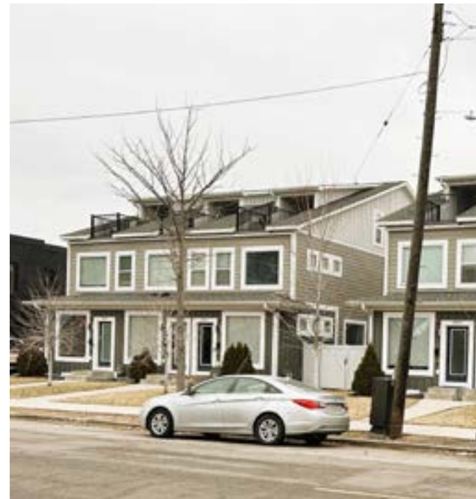
Building size limits ensure buildings within the cluster development are consistent with the intended scale of each built form overlay district.
