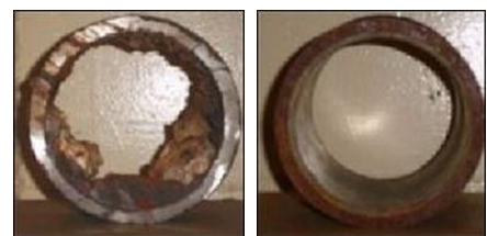
A water main before and after lining
