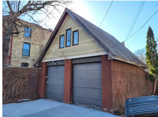
This garage at 108 24th St E uses materials that are appropriate in this district. The walls are clad in brick and lapped siding. The windows are wood and the roof has asphalt shingles.
