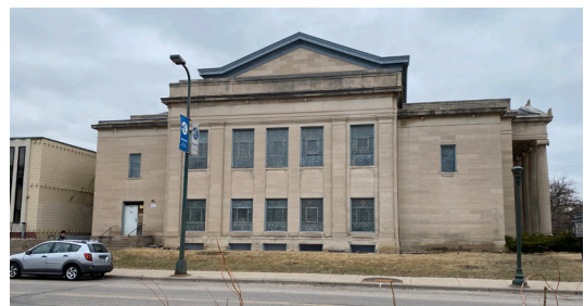
This is the Minneapolis First Seventh-day Adventist Church at 4 24th St E. On the bottom is a view of the west elevation. On the top is an aerial view (Courtesy of MinneAtlas).
