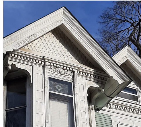
The house at 2429 1st Ave S has many historic wood features. The green lap siding, paneled trim around the windows, and shaped shingles in the gable ends are all original. The gables also have a row of dentils, bargeboards along the eaves, and scroll brackets in the overhang.
