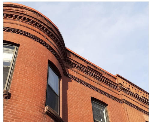
Note the historic brickwork at 100 25th St E. These rowhouses have brick dentils and brackets along the cornice line.
