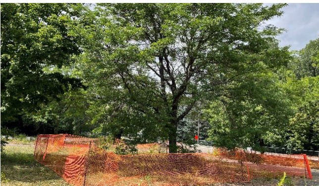
A large tree enclosed by an orange plastic mesh fence to protect it during construction activities. The possibly for protection or construction.
