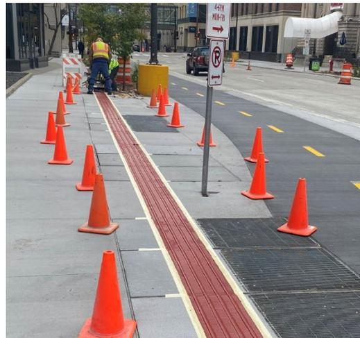
Figure 5: MMA tactile edge being installed on 4<sup>th</sup> St over Xcel Energy vaults
