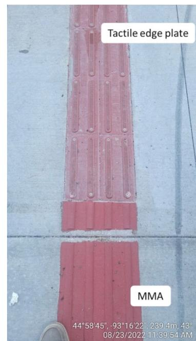
Figure 2: Tactile edge products, plate vs MMA
