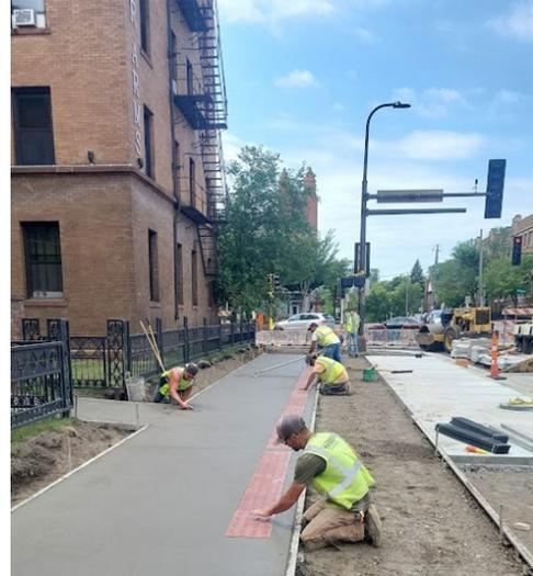
Figure 4: tactile edge plates being installed on Franklin Ave
