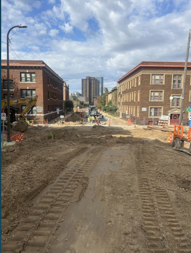
South of I-94 Bridge – Curb and Gutter Install
