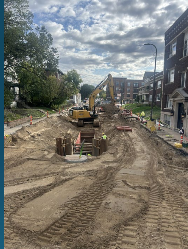
South of I-94 Bridge – Sanitary Sewer Installation
