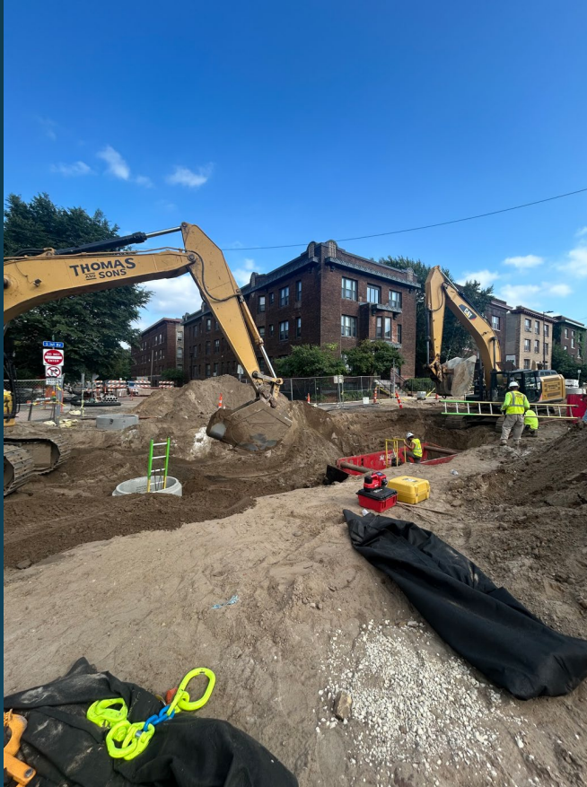
South of I-94 Bridge – Sanitary Installation
