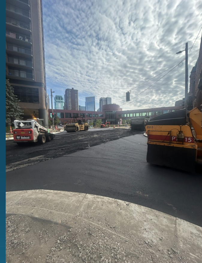
Grant St – Paving
