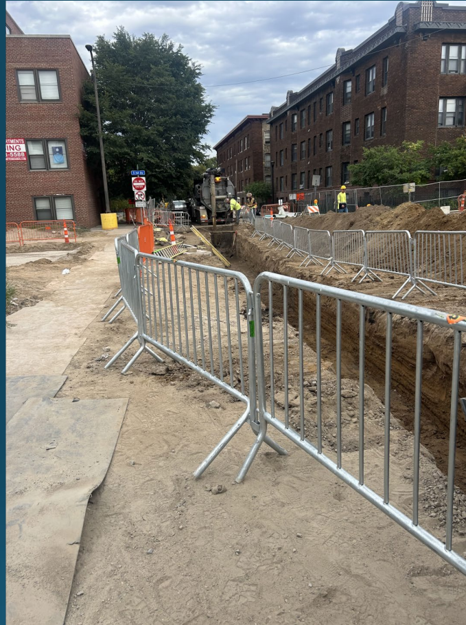
18 th St – Centerpoint Gas Steel Pipe Installation
