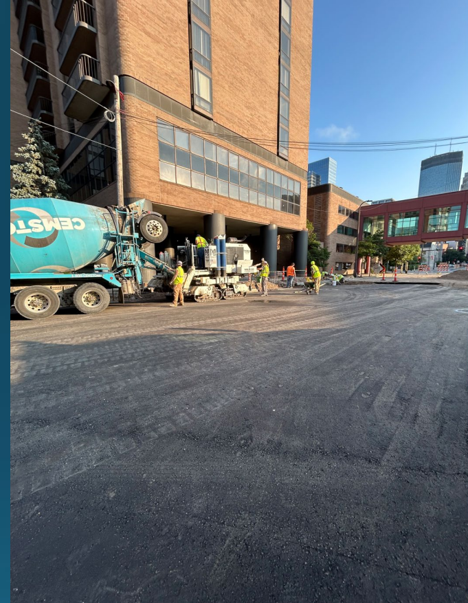
Grant St – Curb and Gutter Install
