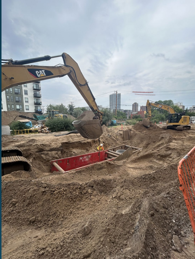
South of I-94 Bridge – Sanitary Installation
