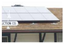
Attach solar collectors to a historic roof in a minimally invasive and reversible manner. In this example the panels are mounted such that the original shingles are saved.
