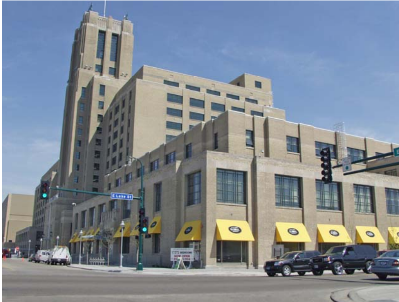
West and south facades, 2006
