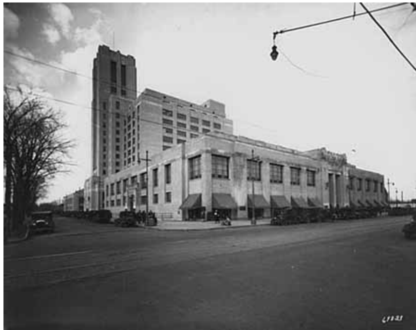
South and west facades, Sears, Roebuck and Company, ca. 1928. Photograph: Minnesota Historical Society
