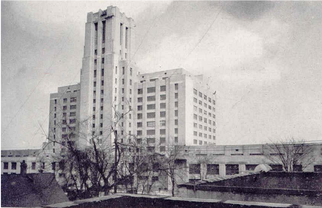
West facade, Sears, Roebuck and Company, ca. 1928. Photograph: Forum , September 1929
