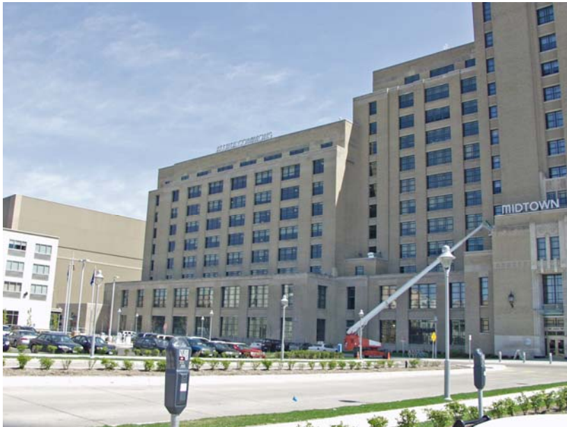
West facade, north end, 2006
