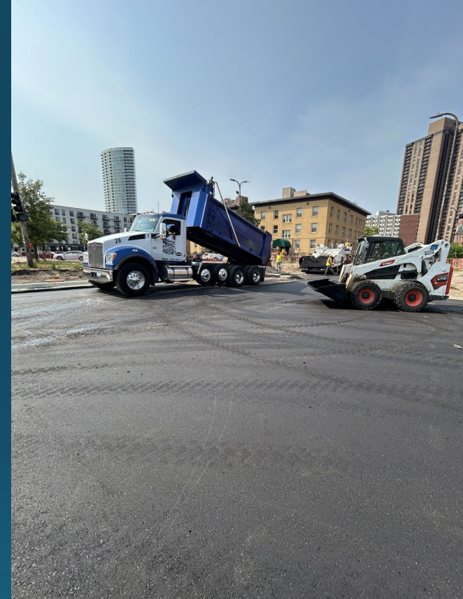
North of I-94 Bridge – Flatwork Installation
