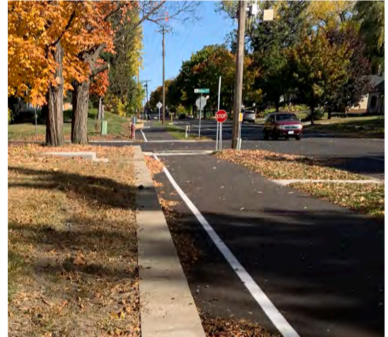
37th Ave NE trail west of Central Ave NE
