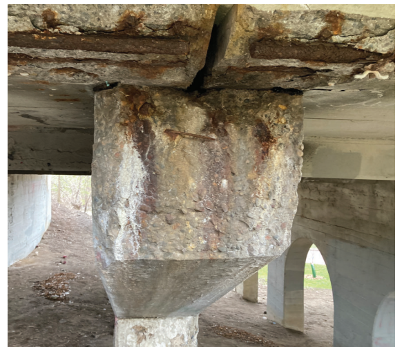
Cracks and Concrete Spalling on Arch Rib
