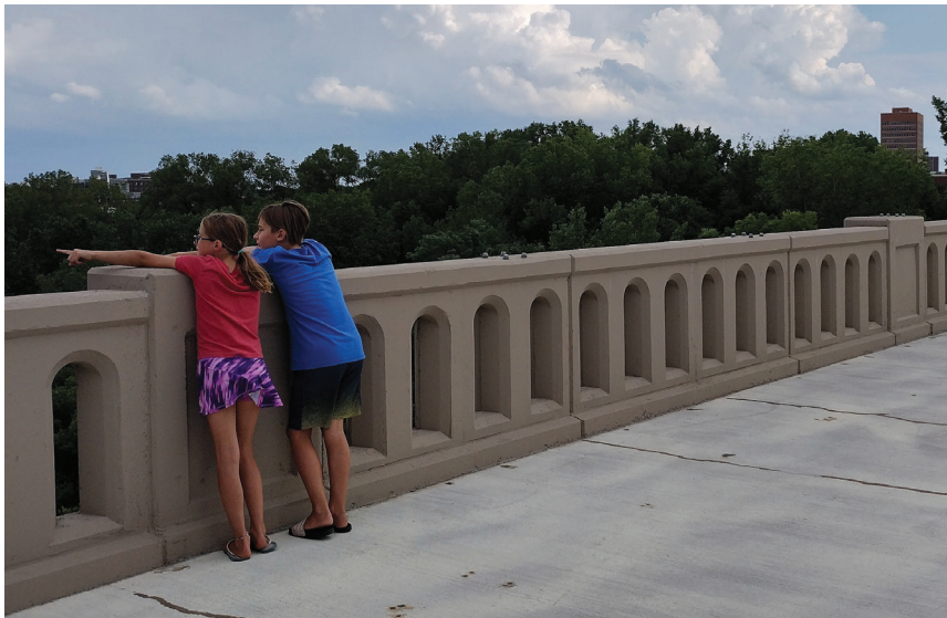
The proposed railing design (similar shown above on 10th Ave bridge) reflects the original design and is used on similar bridge rehabilitation projects in Minneapolis.
