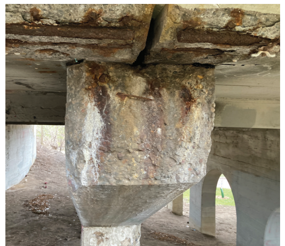
Cracks and Concrete Spalling on Arch Rib
