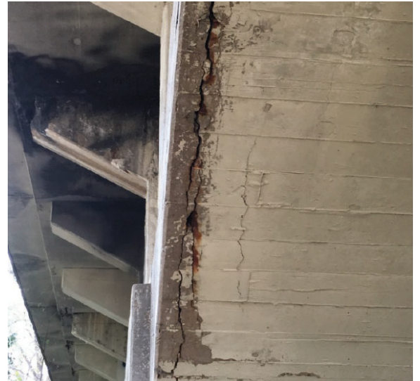
Cracks and Concrete Spalling on Arch Rib
