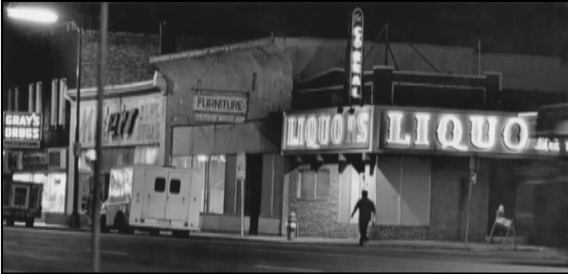
FIGURE 26. VIEW OF 1401-1413 E FRANKLIN AVENUE, UNDATED
