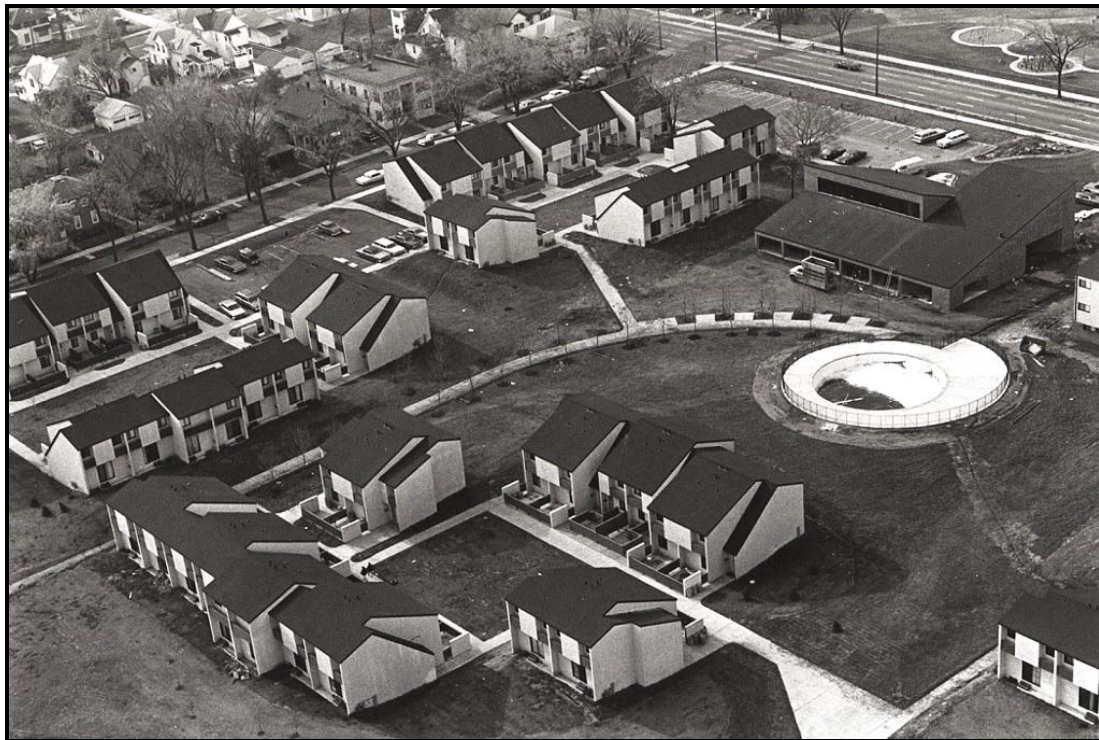
FIGURE 32. AERIAL VIEW OF LITTLE EARTH IN 1973
