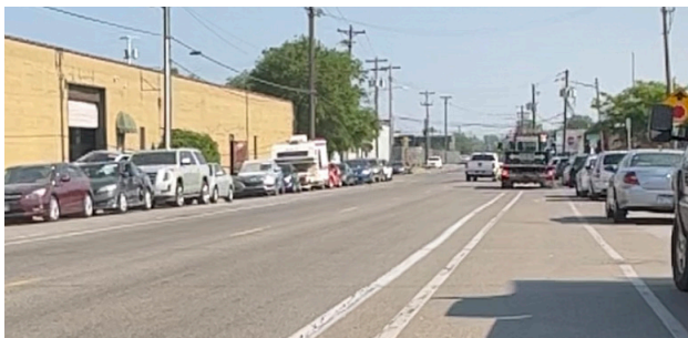
Existing Conditions– North 2nd Street
