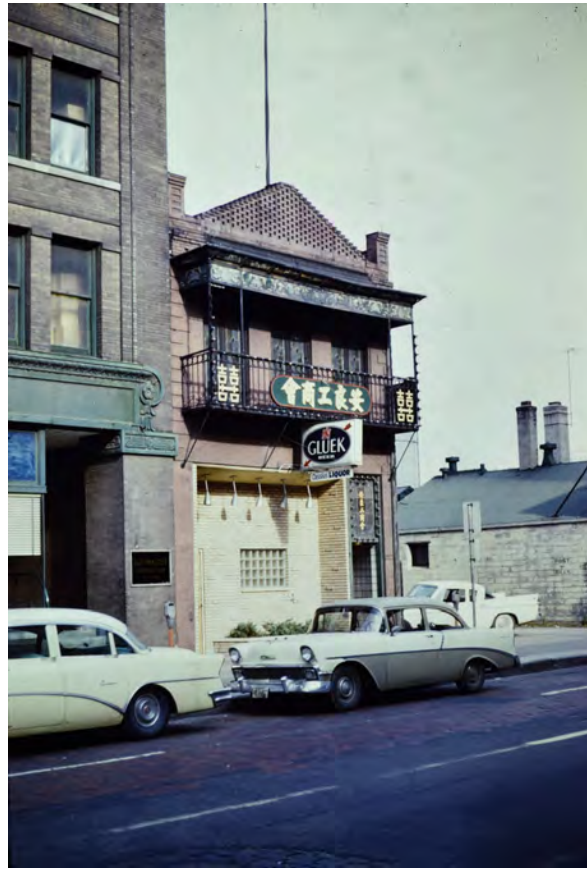
221_Cassius Bar_Hennepin County Library 318 3rd Street South (non-extant)
