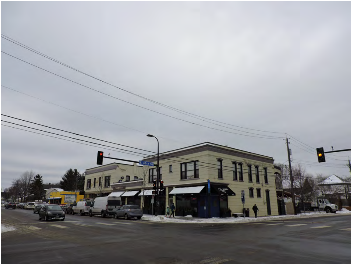
38th Street East & Nicollet Avenue_Facing Northeast
