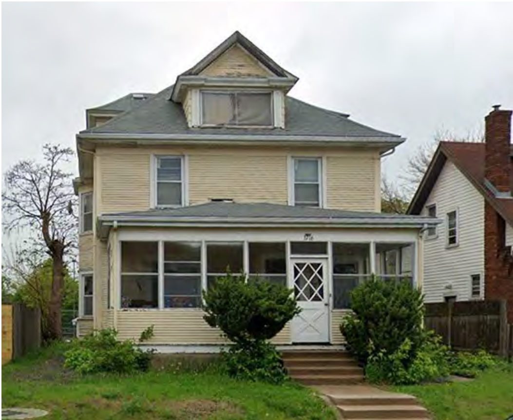
29_Solomon Hughes, Sr. House_Google 3716 4th Avenue South
