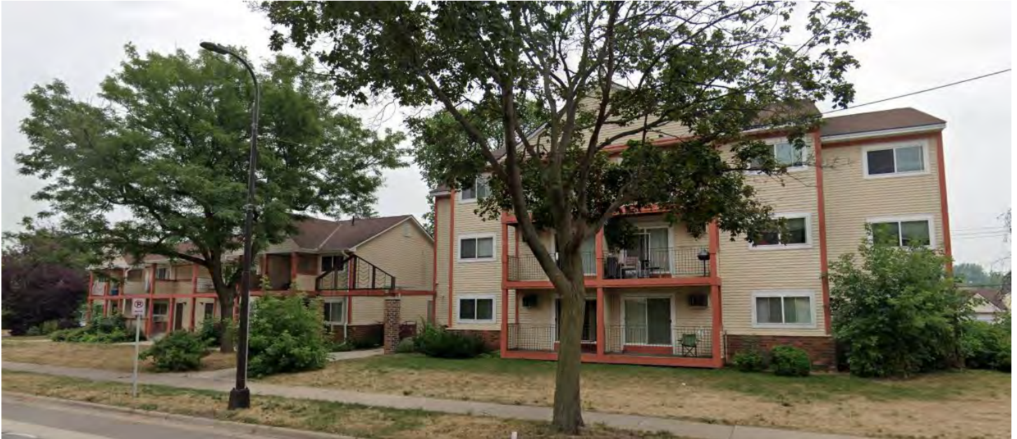
143_Apartments & Townhouses_Google 1701 Plymouth Avenue North
