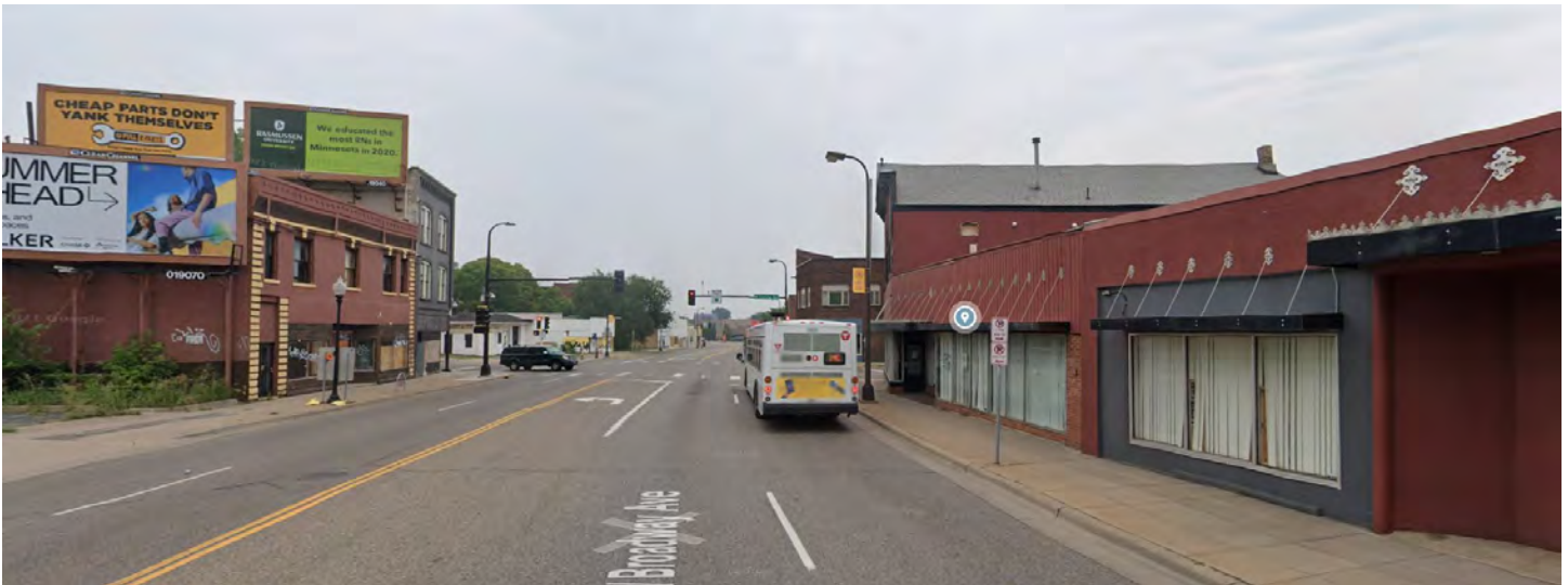
West Broadway and North Penn Commercial Area (HE-MPC-12102), at Irving Avenue North_Google
