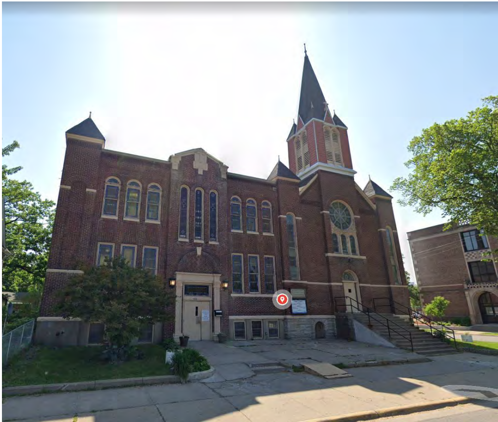
159_Greater Mt. Vernon_Google 1800 DuPont Avenue North
