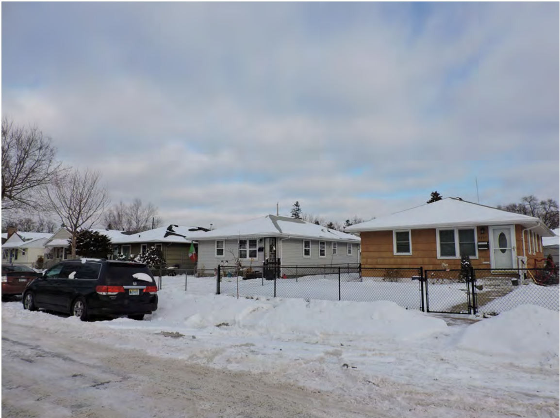
Tilsenbilt Homes Historic District 4th Avenue South & 5th Avenue South, between 39th and 47th Streets East
