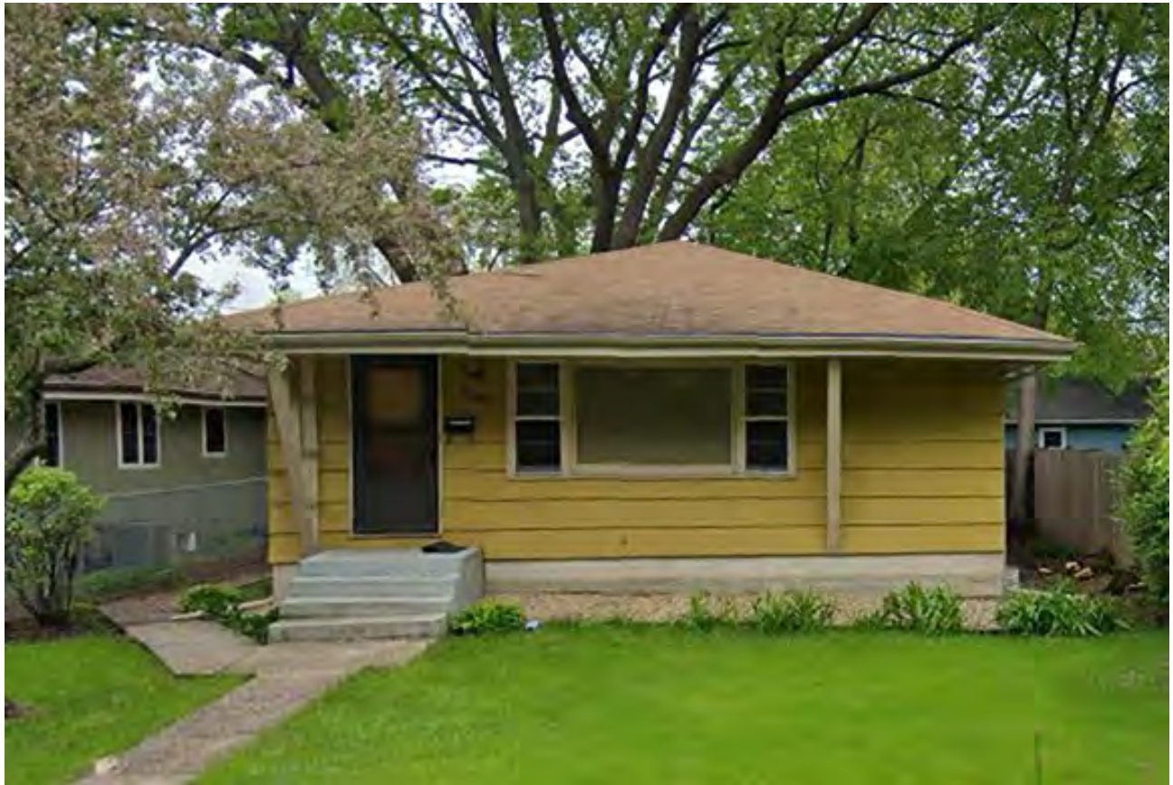
206_Archie Givens House_Google 4248 3rd Avenue South
