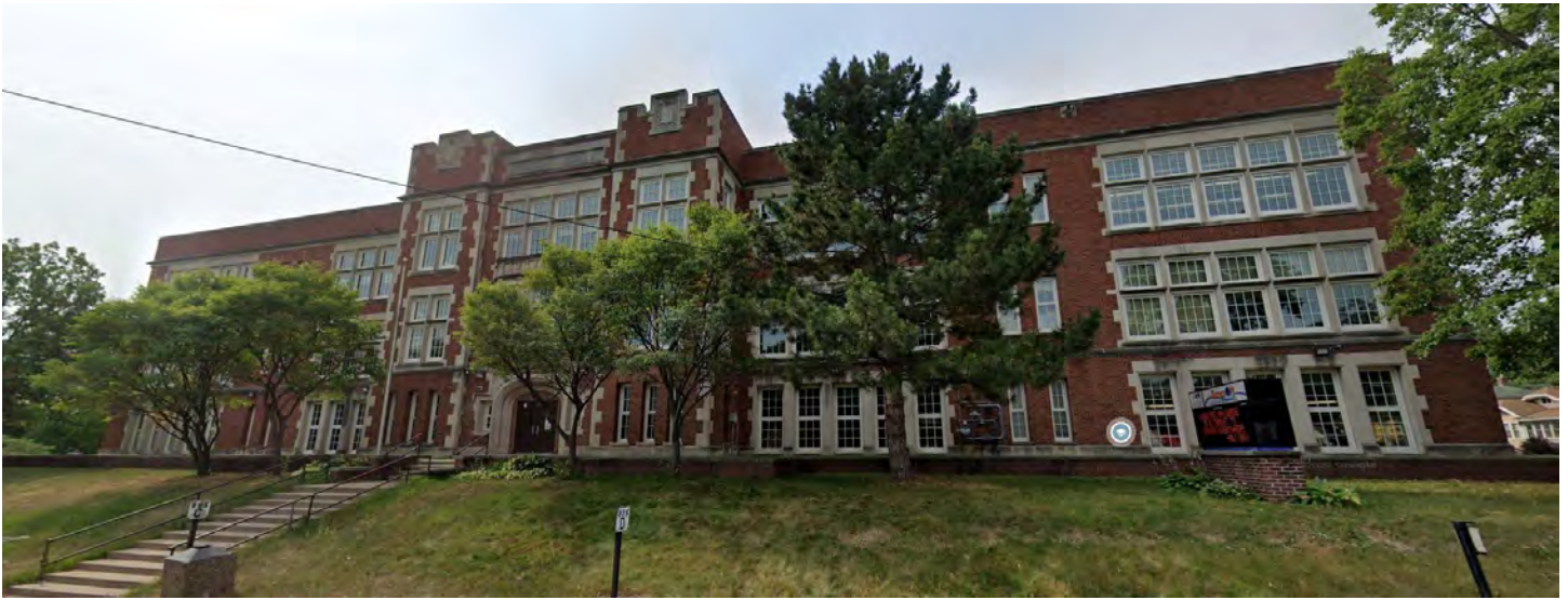
20_Bancroft Elementary School_Google 3829 13th Avenue South (HE-MPC-4691)
