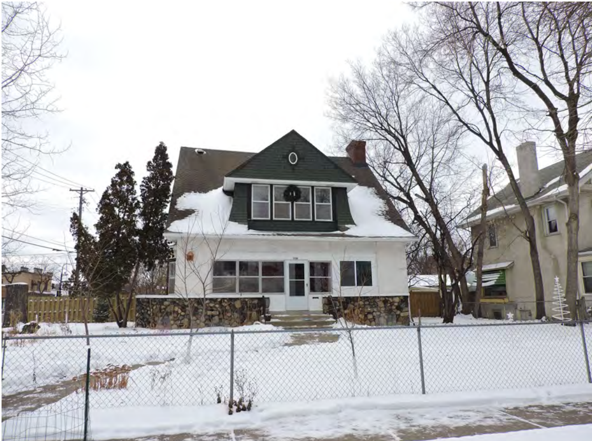
184_St Peter's AME Parsonage (former) 3756 5th Avenue South
