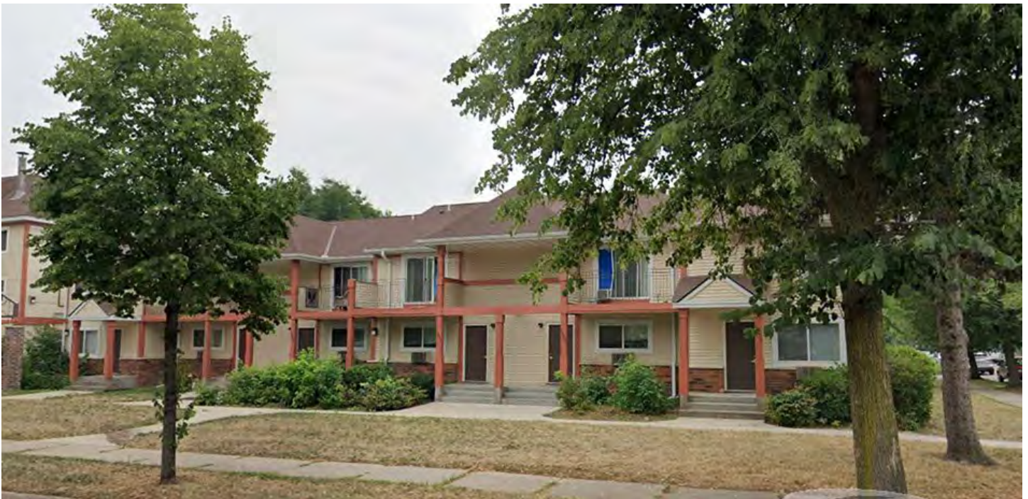
144_Apartments & Townhouses_Google 1815 Plymouth Avenue North
