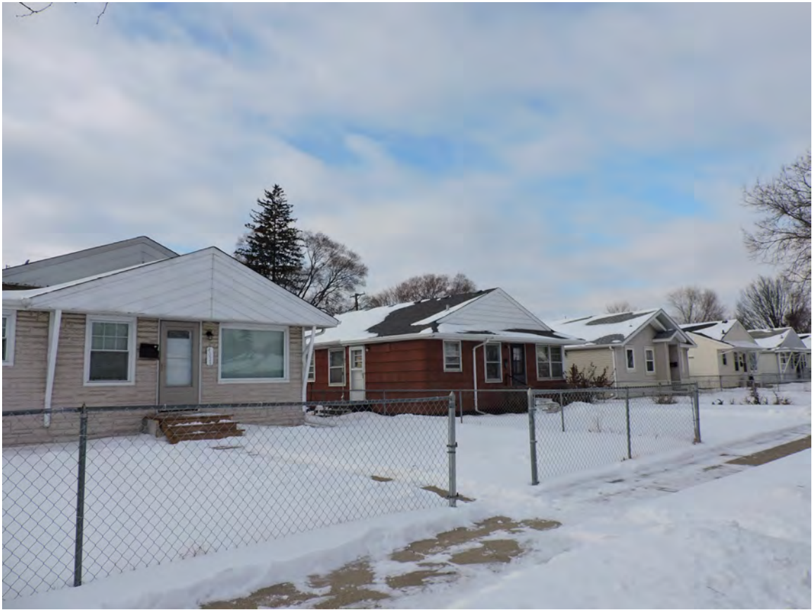
Tilsenbilt Homes Historic District 4th Avenue South & 5th Avenue South, between 39th and 47th Streets East
