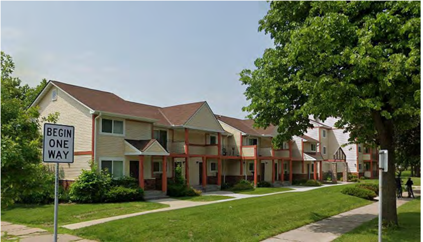
141_Apartments & Townhouses_Google 1501 Plymouth Avenue North
