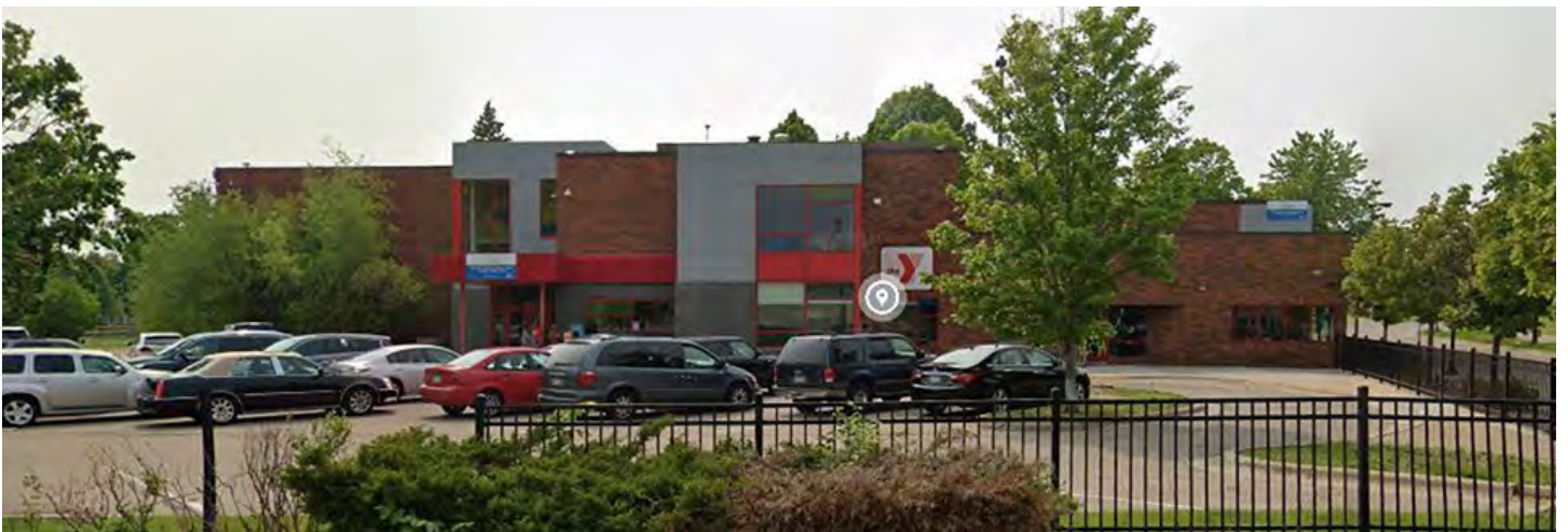
164_North Community YMCA_Google 1711 West Broadway Avenue
