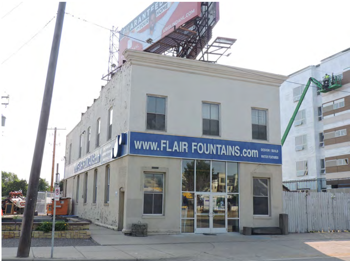
10_Fire Station 24 4501 Hiawatha Avenue (HE-MPC-7413)
