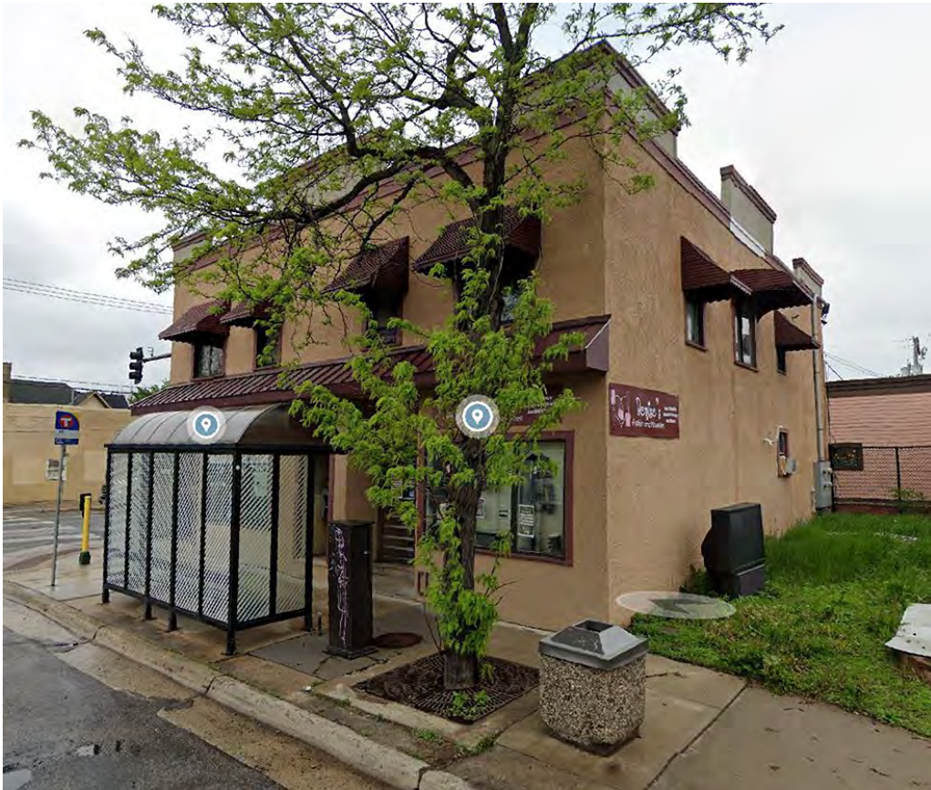
30_Jet Records (right) and 231_Commercial Building (left)_Google 3803 4th Avenue South (HE-MPC-4400, right) and 3801 4th Avenue South (HE-MPC-4399, left)
