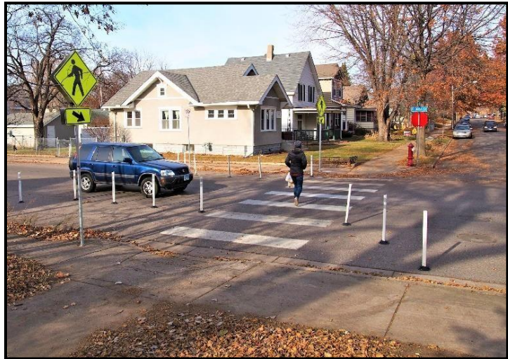
Figure F-5. Temporary Curb Extensions
