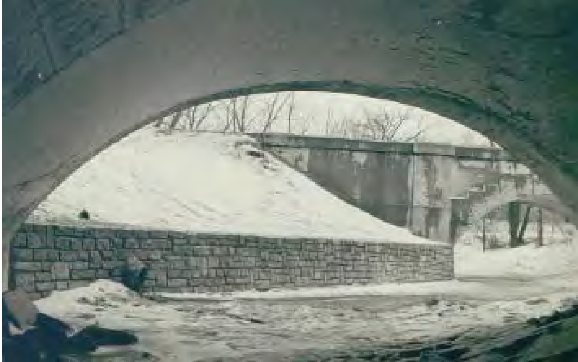
Figure 2.6 Retaining walls along Minnehaha Creek were constructed by the WPA and are characteristic of the types of infrastructure projects that the WPA constructed throughout Minneapolis and the country at large. Retaining walls along Minnehaha Creek, c. 1938. Walter B. Dahlberg, The Story of W.P.A. in the Minneapolis Parks, Parkways, and Playgrounds for 1938 ([Minneapolis, MN?]: Board of Park Commissioners, 1939).
