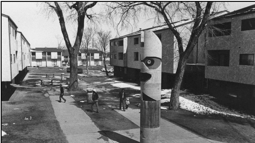
Little Earth of United Tribes - Example of Housing Units, c.1973 View to Northeast from North of Housing Office (Little Earth of United Tribes 2016)
