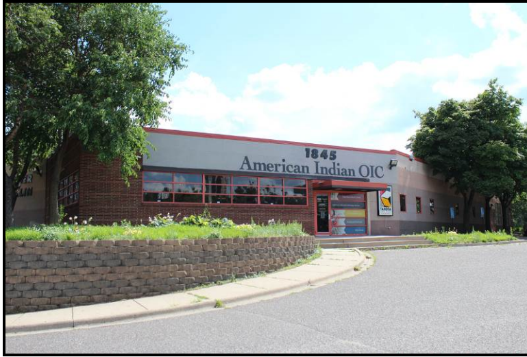
American Indian Opportunities Industrialization Center 1845 E Franklin Avenue, View to South
