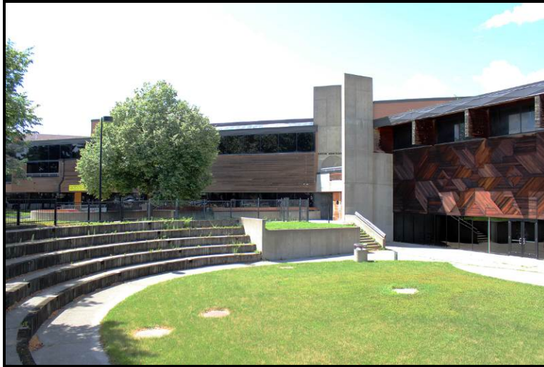
Minneapolis American Indian Center 1530 E Franklin Avenue, View to West
