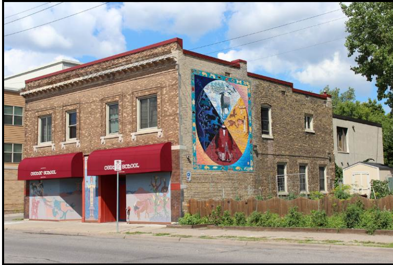
Nawayee Center School 2421 Bloomington Avenue S, View to Northeast
