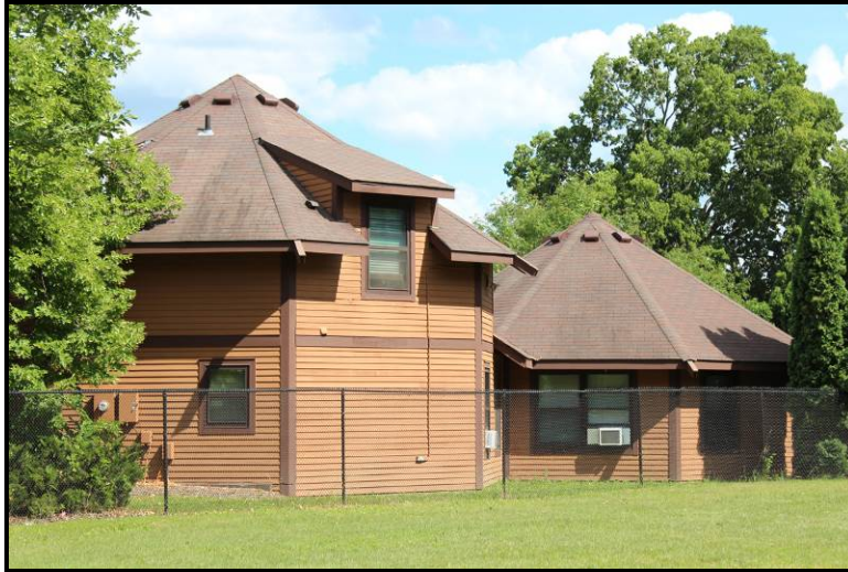
Maynidoowahdak Odena (Representative) 1321 E 23 rd Street, View to Southeast
