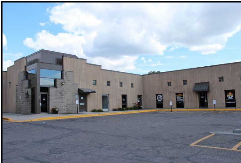
Franklin Business Center 1433 E Franklin Avenue, View to Southeast
