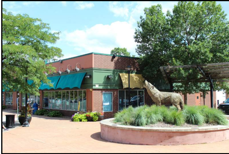
Franklin Circles Shopping Center 1221 E Franklin Avenue, View to Southeast
