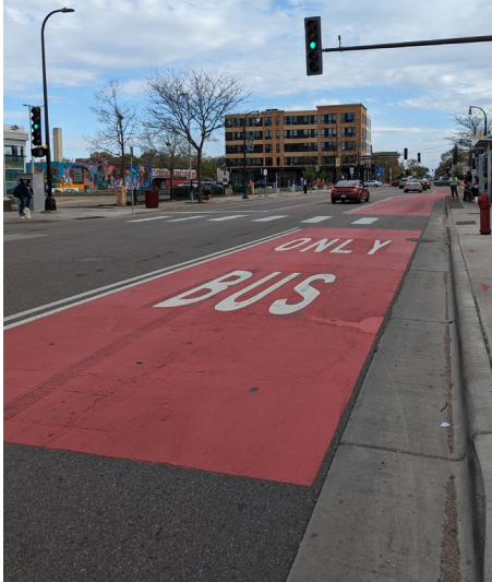
Figure 18: The paint on Chicago Ave showing some chipping and tire staining
