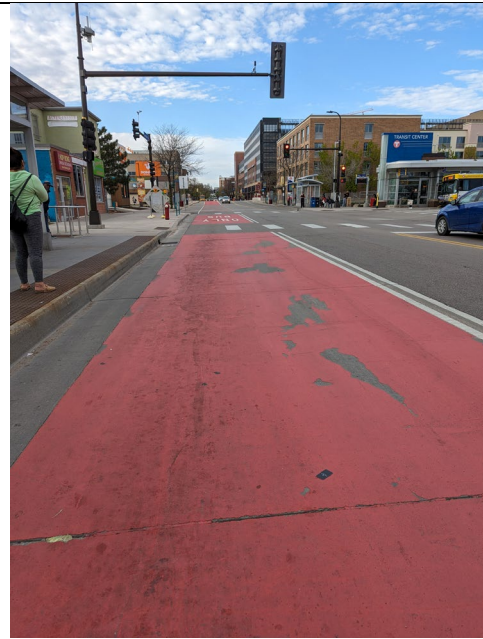
Figure 12: Flaking seen at the Chicago Ave & Lake St bus stop
