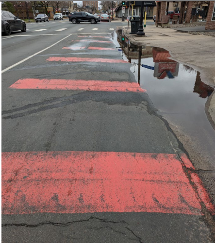
Figure 13: Dashed area degradation and pavement damage seen next to the Hennepin Ave & W 24 th St bus stop and adjacent driveway
