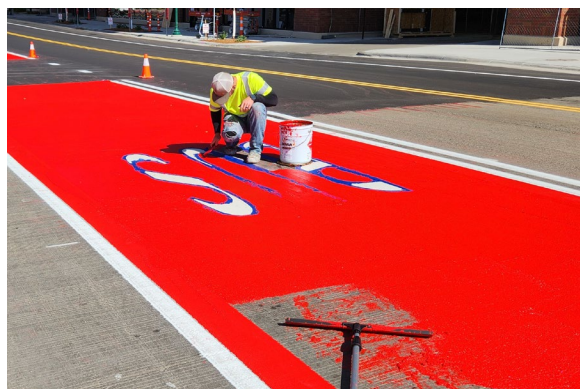
Figure 3: Crews applying MMA by hand on the main lane sections on Chicago Ave (September 2022)
