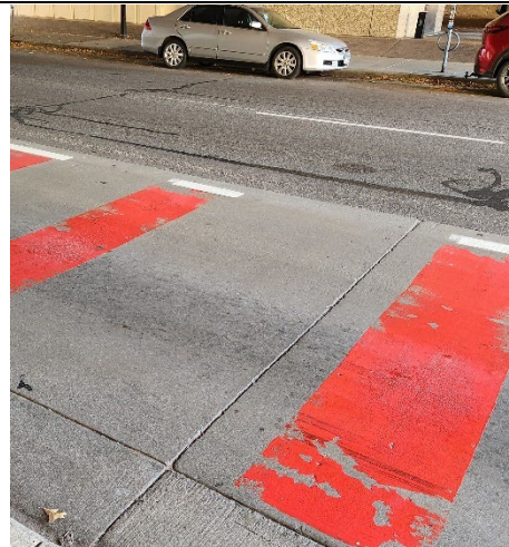
Figure 14: Dashed area degradation seen at Park & 7 th bus stop on 7 th St.
