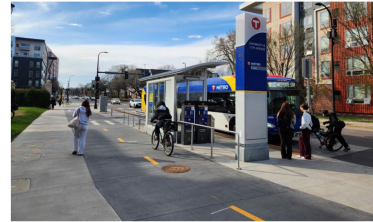
Sidewalk-level protected bike lane, wrapped around BRT platform
