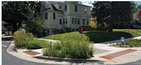
Curb extension & pedestrian ramps
