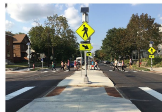
Median with flashing beacon
