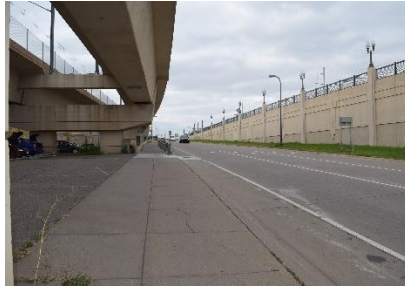
Southbound Hiawatha Avenue Exit Ramp, before metal in-concrete fence (Looking North)
