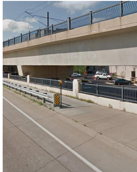
In-sidewalk metal fence/guardrail
