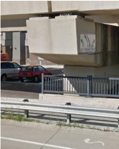
Low bridge deck
