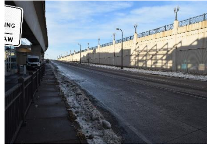
Southbound Hiawatha Avenue Exit Ramp at Lake Street (Looking North)
