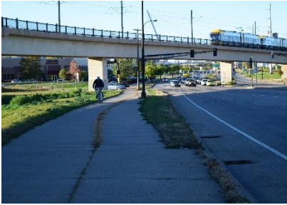
Hiawatha Avenue west sidewalk and shoulder at 28 th Street (Looking North)
