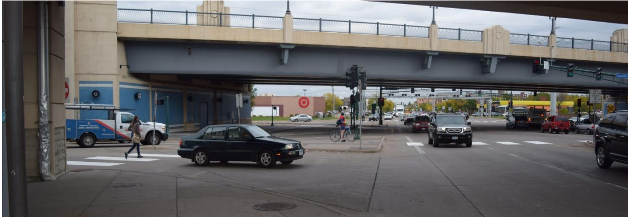
Figure 2-10: Bicyclist waiting on the island to cross Lake Street
