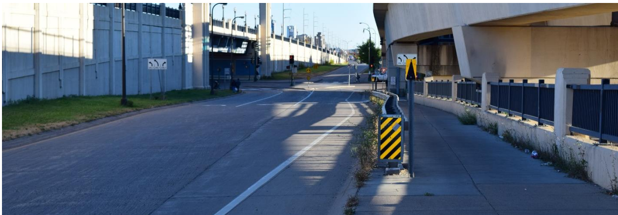
Figure 2-11: Southbound approach to Lake Street from bicyclist's perspective
