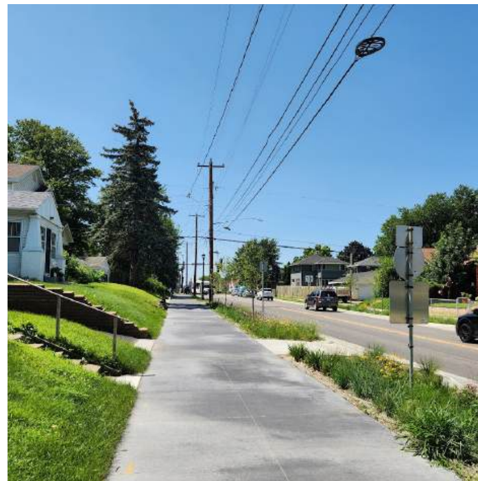
Example: Shared Use Path and green stormwater facility along Dowling Ave in North Minneapolis. This is what 38th St would look like in the recommended design.
