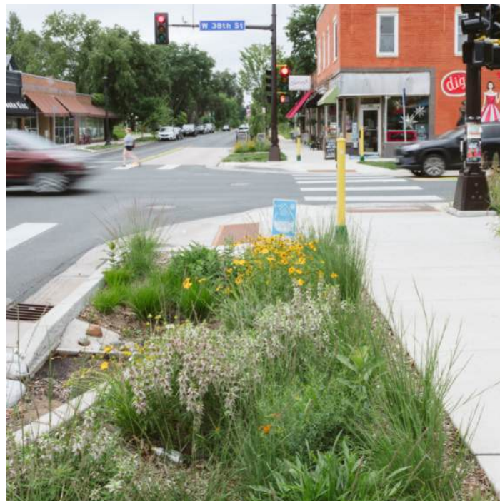
Example: Green stormwater facility at 38th St and Grand Ave.
