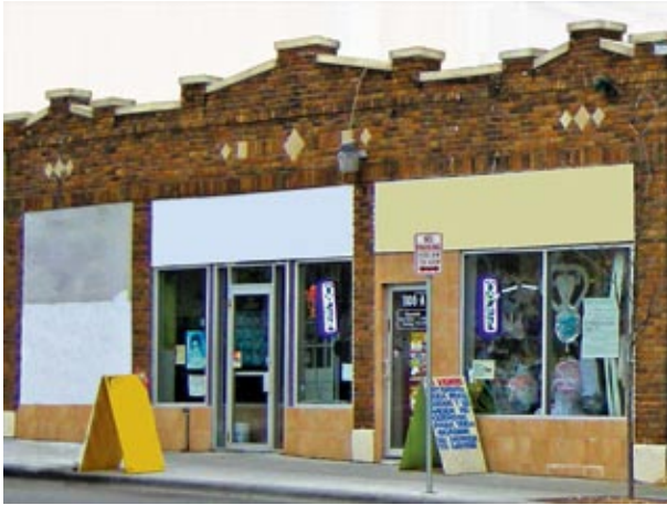
BEFORE Covering windows and skirtboard panels with boards or other materials is discouraged.
