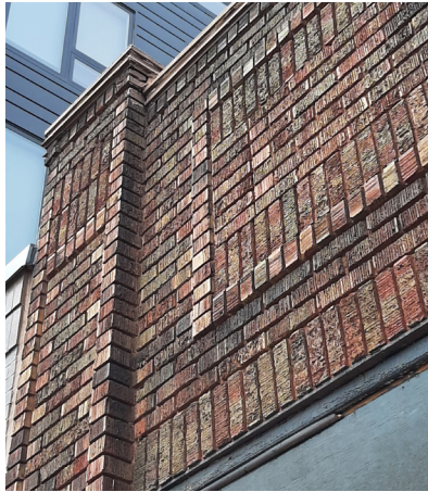
Masonry is a common wall material throughout the district. Notice the different bond patterns. This wall has stretcher bond, soldier courses, header courses, and stacked bond.
