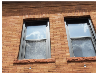
These replacement metal windows at 1401-1411 4th St SE are set within the historic openings. The jack arches above and sills below are original.
