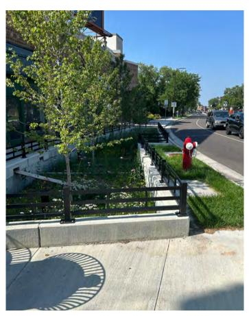
Crews are adding about 70 stormwater BMPs (Best Management Practices). These are special features that catch, hold, and infiltrate rainwater rather than flowing directly into lakes or rivers. These features also make us more resilient to climate change, provide pollinator habitat and reduce the urban heat island. This project includes:
