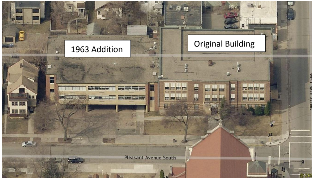
FIGURE 3. MOYNIHAN HALL, EASTERN ELEVATION, APRIL 1, 2015, CONNECTEXPLORER AERIAL IMAGE DATABASE.
