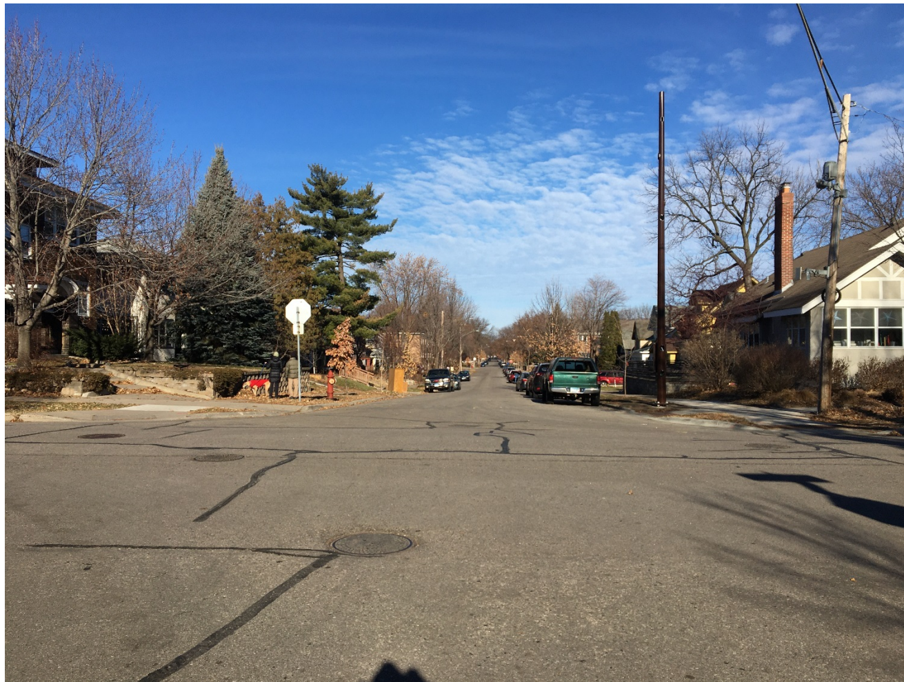
Figure 7: Looking north on Aldrich Ave S at 40 th St W. This crossing is 36 feet wide. For comparison, Public Works is proposing narrowing crossing distances on Bryant Ave S to 22 feet in the Bicycles on Bryant option.
