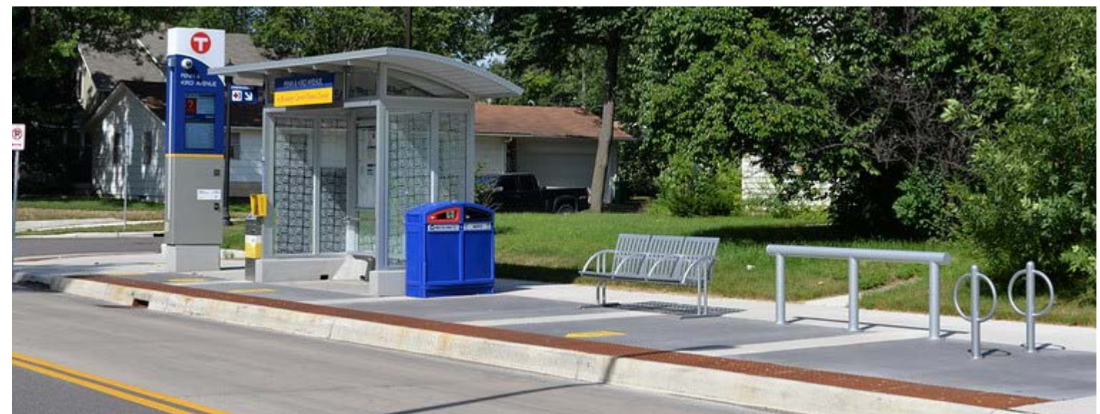
Figure 6: C Line BRT station platform
