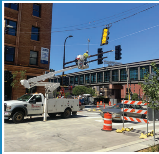
Signal system installation at the 2nd Ave. N intersection.
