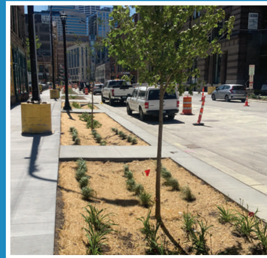
Completed landscaping between 2nd Ave. N and Hennepin Ave.
