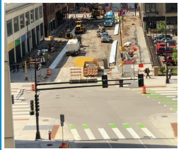
Roadway reconstruction near the Hennepin Ave. intersection.
