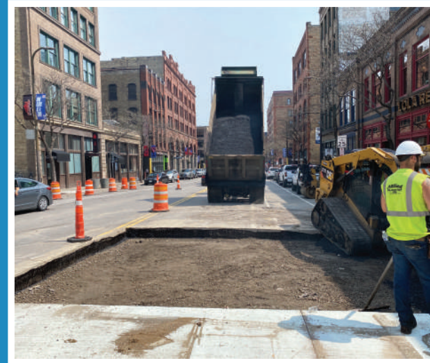
Roadway repaving at the 1st Ave. N. intersection.
