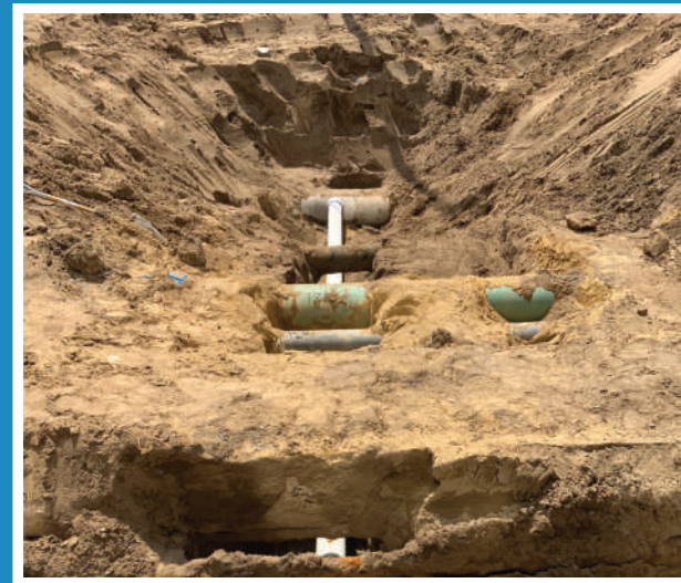
Mainline storm sewer and building rain leaders connections
