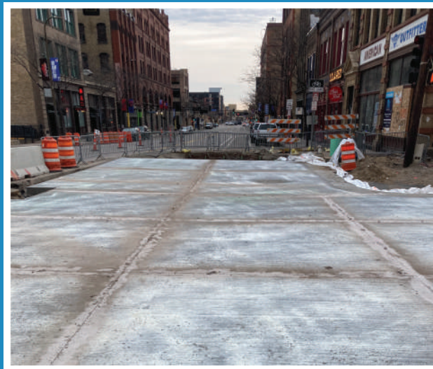
Newly paved northbound lanes on the 1st Ave intersection
