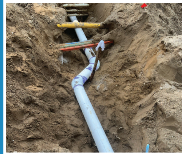
Final rain leader hook ups east of 1st Ave. N
