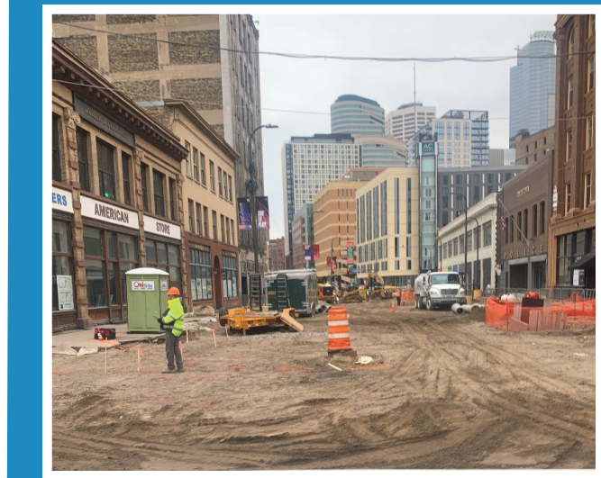
Roadway reconstruction underway on 4th St. near Hennepin Ave.
