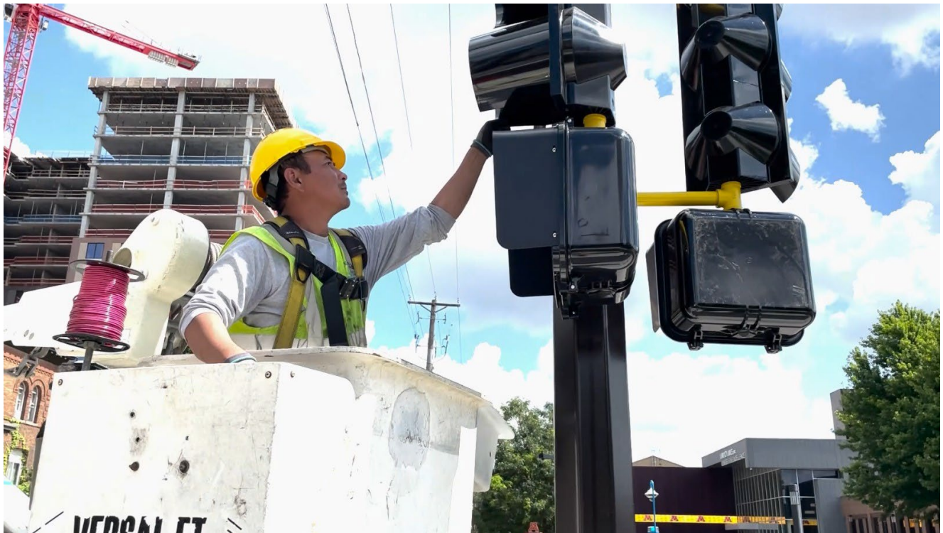
Theun Keosaksith installs a new traffic signal light
