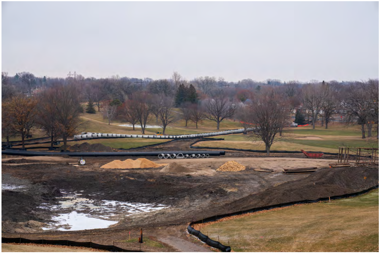
Columbia Golf Course project under construction
