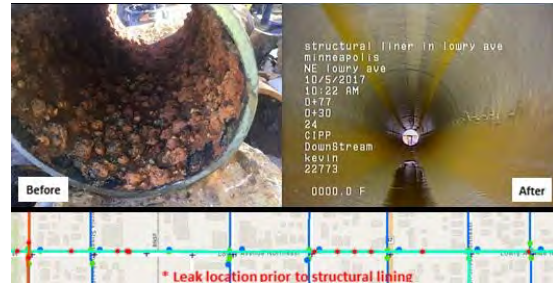
Inside of a water main before and after structural lining.
