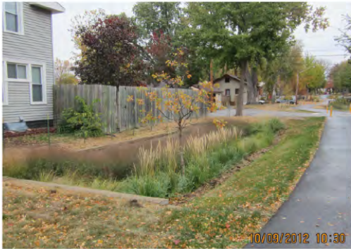
Rain gardens along the completed 37th Ave Greenway provide water quality benefits. Flood storage is located under the mixed-use trail.
