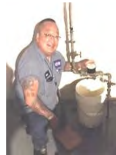
Replacement of a customer's water meter.
