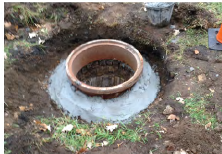
Infiltration & Inflow Repairs
