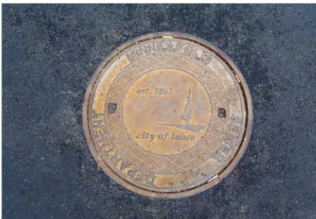
Manhole Cover Replacement
