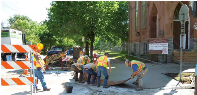
City crews install a new, ADA-compliant pedestrian ramp.
