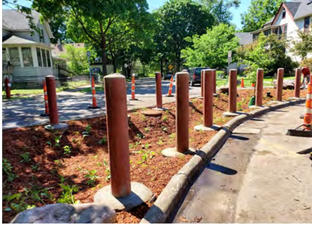
Talmage Diverter Green Infrastructure Project: just after planting
