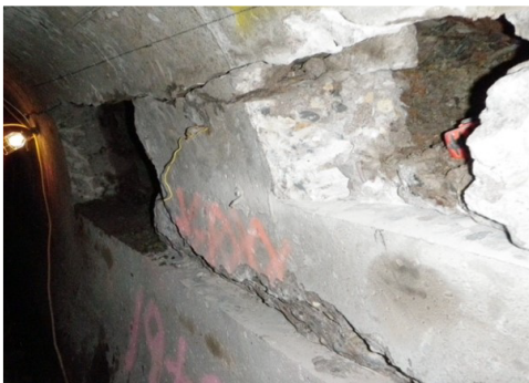
Deterioration in tunnel
