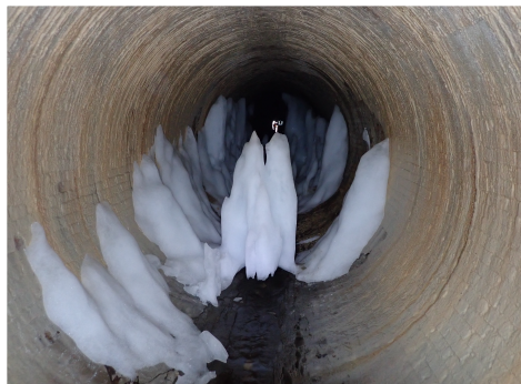
Ice buildup in tunnel
