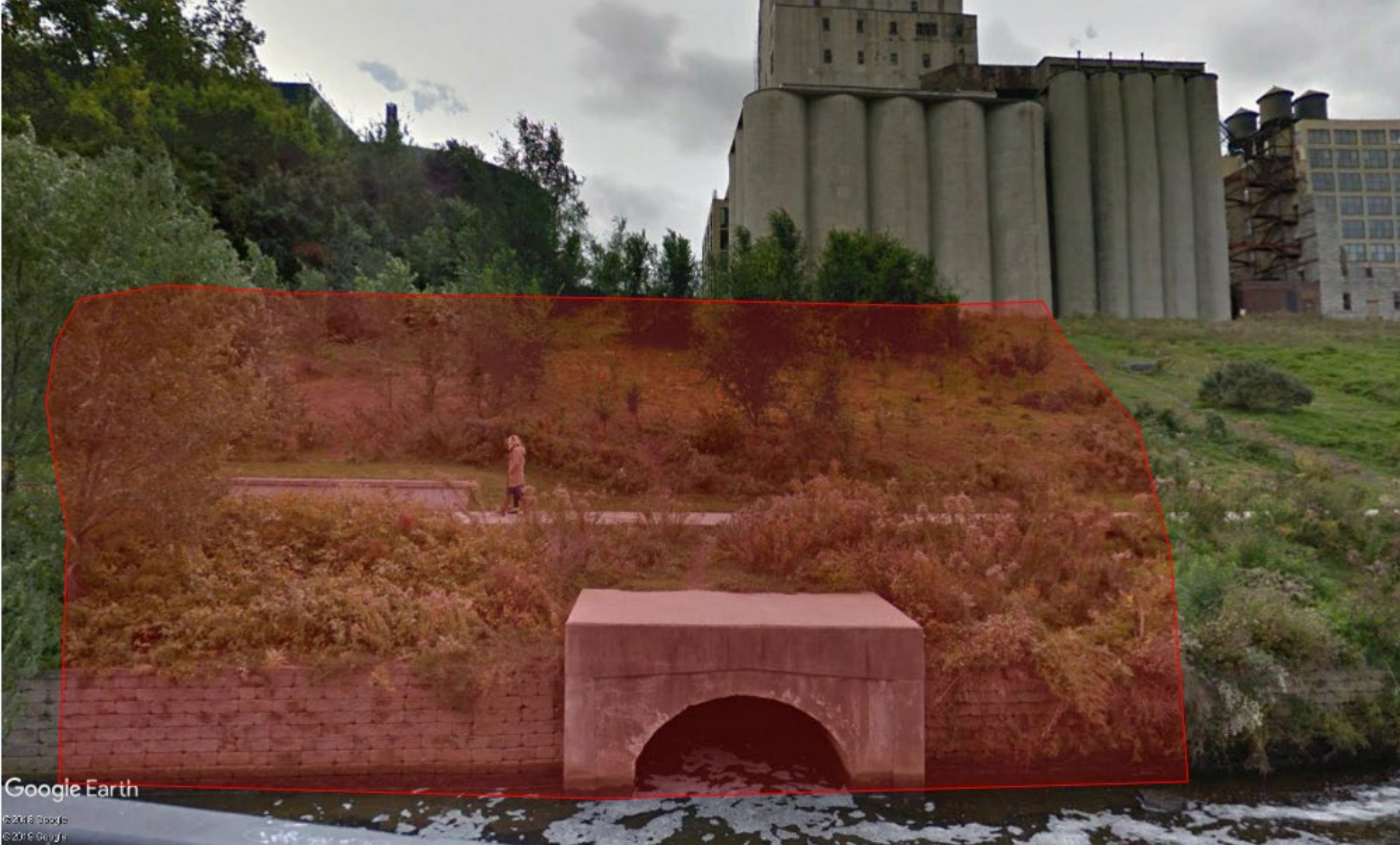
Outlet Excavation Area
