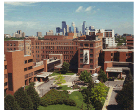
Abbott Northwestern Hospital in South Minneapolis
