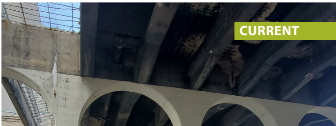
Bridge deterioration and removal of sidewalk
