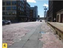
4 If vertical dimension is greater than 30 inches, railings may be required to meet current building codes
