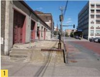
1 Existing stairs at loading dock in poor condition
