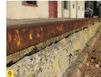
9 Concrete is deteriorating at edge of dock
