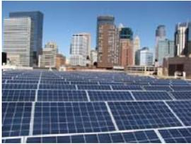
The Upper Midwest's largest solar photovoltaic system is now under construction at the Minneapolis Convention Center, with 1,250 of its 2,613 solar panels installed.
