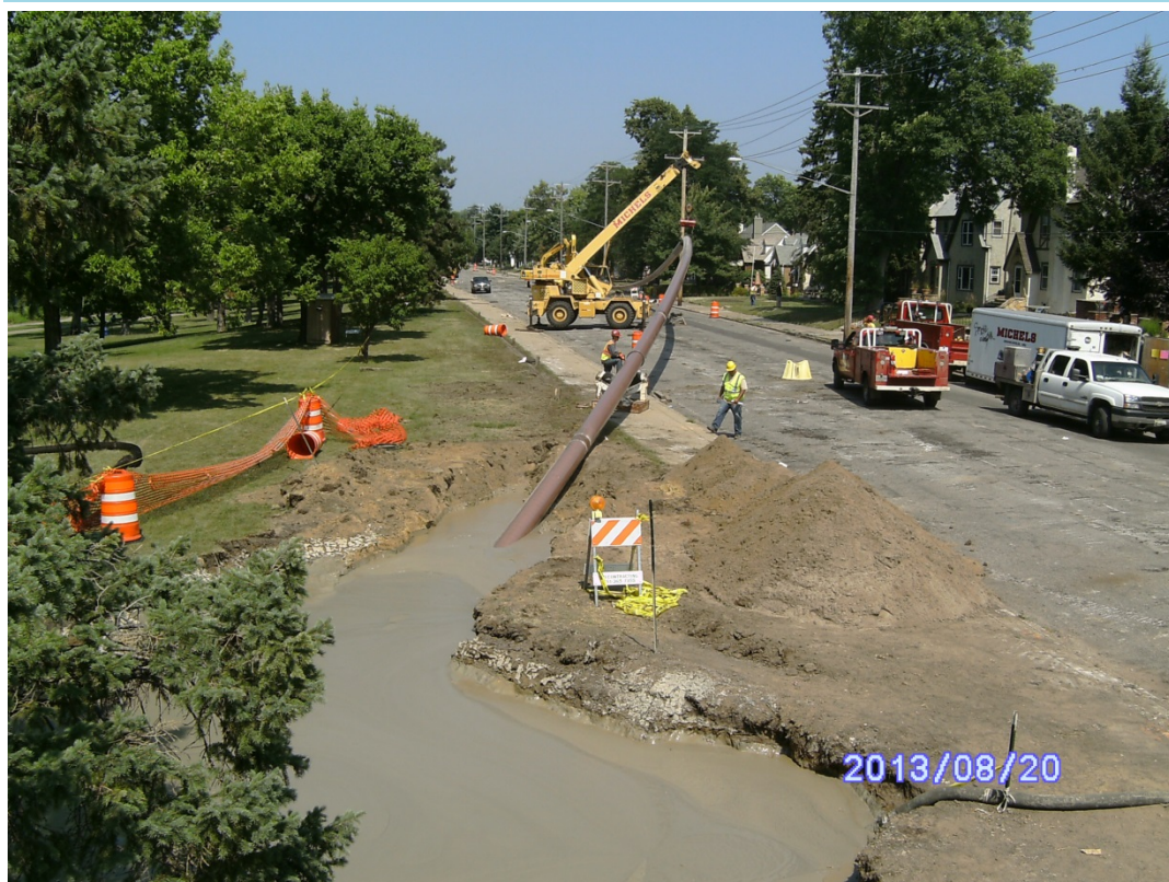
CenterPoint crews installing a gas main that runs 60 feet below the creek.
